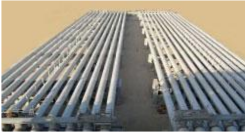
Figure 19.2.1. Finger slug catcher.
