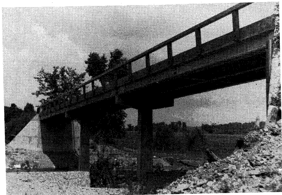
Fig. 18. Cheatham County Bridge of three 50-ft (15.3 m) spans made continuous by reinforcing in composite pour over supports. Pier caps are precast. Built in 1955.
