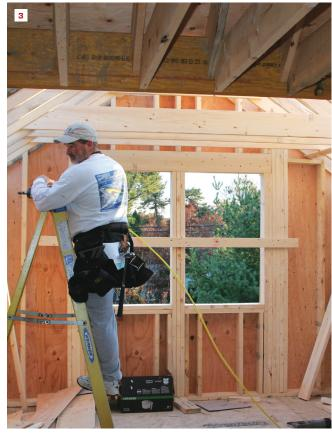
however, function as both a rafter tie and a ceiling joist.
