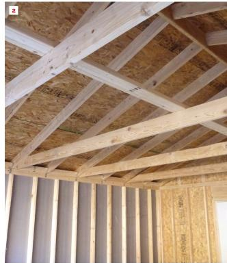
ceiling below without an attic space (although the code does allow for building an attic by adding properly sized ceiling joists). The ridge-beam approach is simple except for the sizing of the beam, for which the IRC does not provide guidance. Using an engineered beam (such as an LVL) for the ridge is helpful in this regard because large spans can be achieved and span tables are usually available from the manufacturer.
