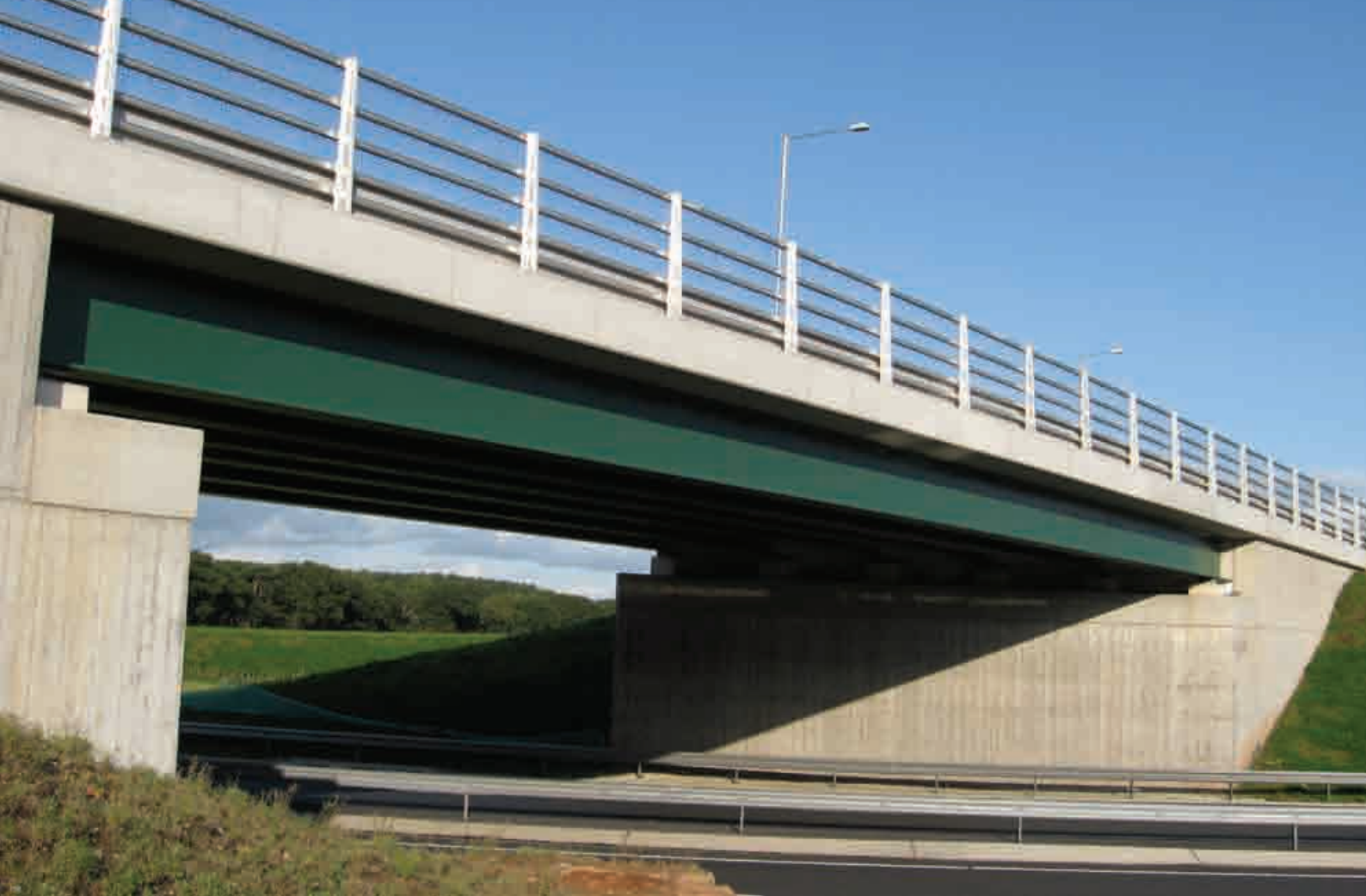
Above: A1 Appleyhead – Typical highway bridge with S355 steel
