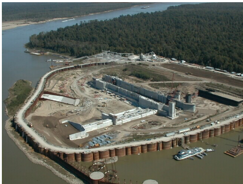
Figure 2. Cofferdam at Montgomery Point Lock, USA (Courtesy: U.S.Army Corps of Engineers 2004)
