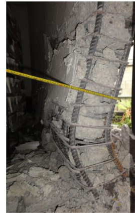
Figure 3-3 – Wall buckling, 2011 Christchurch earthquake.
