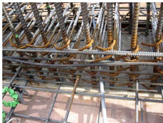
Figure 7-2 – Boundary confinement for planar wall.
