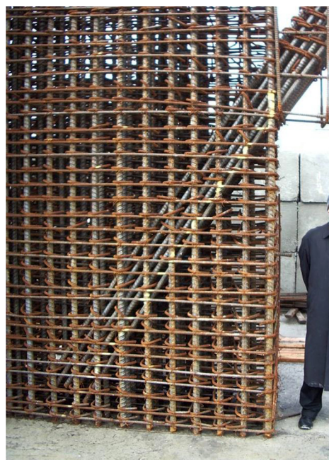
Figure 7-4 – Anchorage of diagonal reinforcement in heavily reinforced boundary element.
