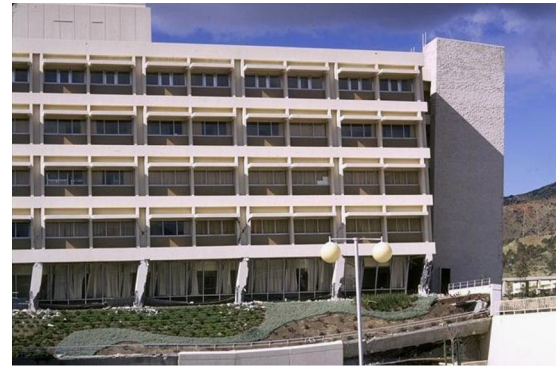
Figure 2-4 – Weak story damage, 1971 San Fernando earthquake.
