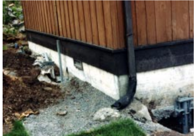
Twelve screw anchors were installed on the outside.
