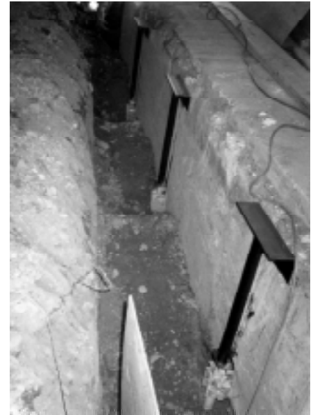
Pipe and flange assembly was welded onto the underpinning bracket's T-pipe to give added bearing area for the new 7" structural slab
