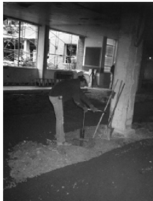
Fabricated cap with bolt allowed for precise adjustment with a laser level providing a reference point
