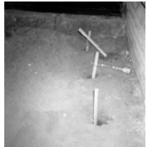
Threaded stud adapter (on ground) will be attached to the screw anchors and lateral anchors. A square plate will be double-nutted onto the adapter and cast in concrete.
