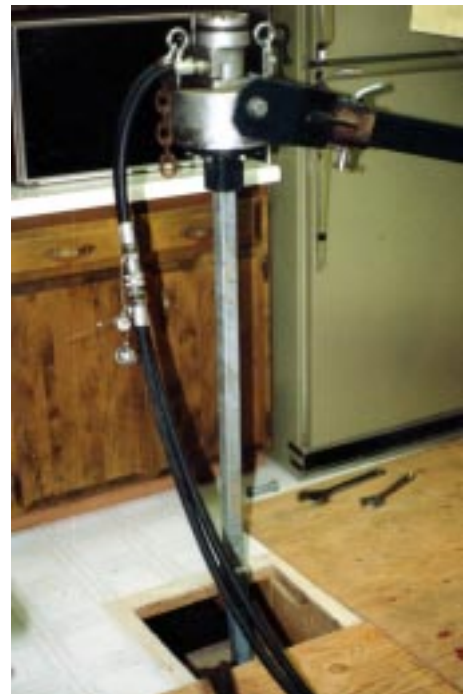
Portable hydraulic driver installing screw anchor through kitchen floor →
