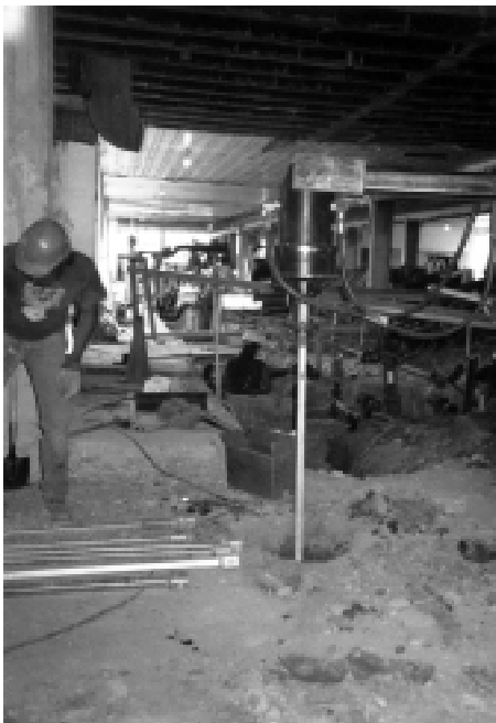
Chance anchor being installed in slab area on a 10' grid
