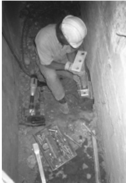
Underpinning bracket being assembled onto Chance HELICAL PIER® Foundation Systems anchor and under utility vault
