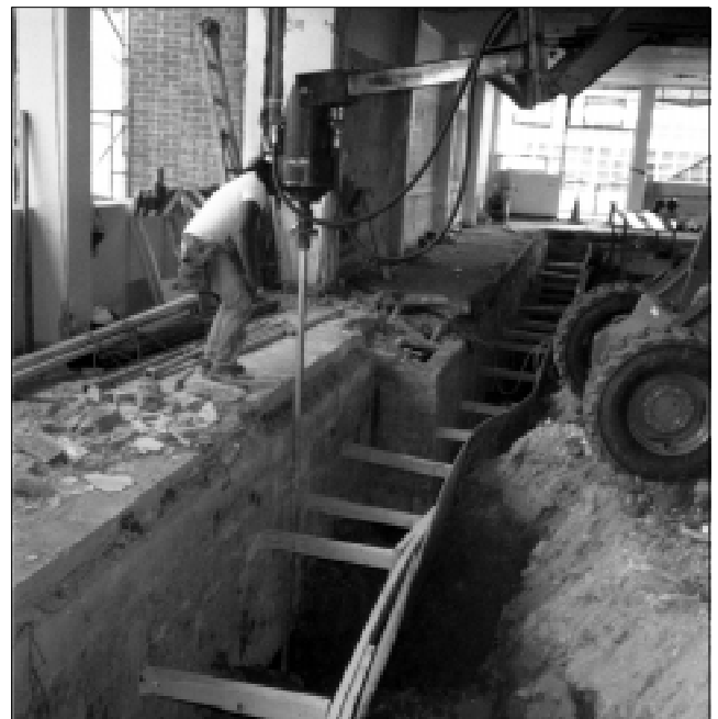
5,000 ft.-lb. hydraulic drive attached to skid loader installs screw anchor along side a utility vault
