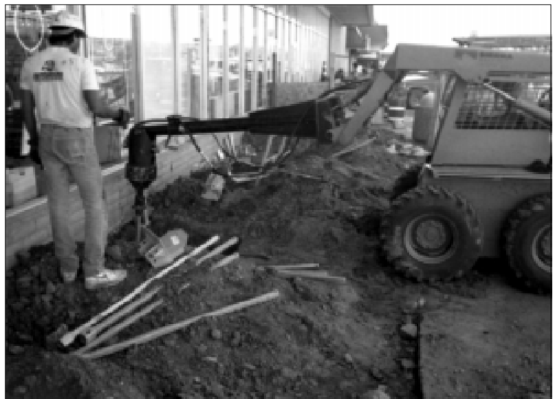
Skid loader driving screw anchor to 40'
