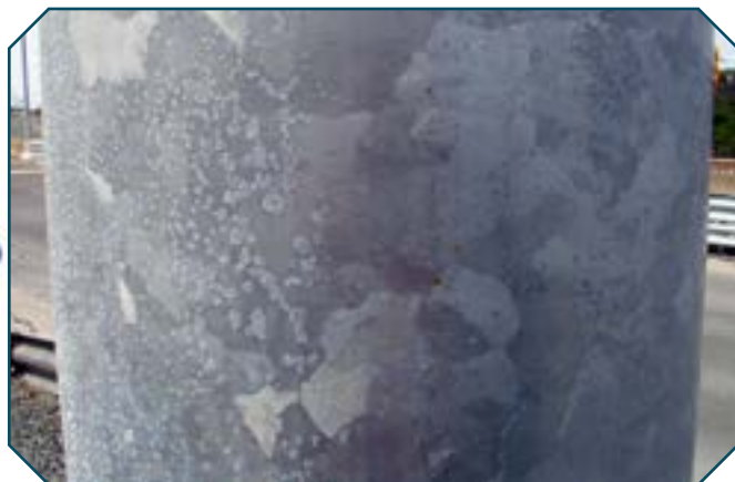
Figure 7: Light wet storage stain
