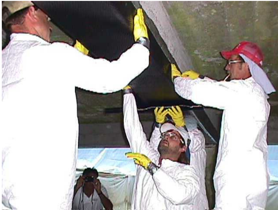
Figure 2.4.1 FRP being installed for strengthening.
