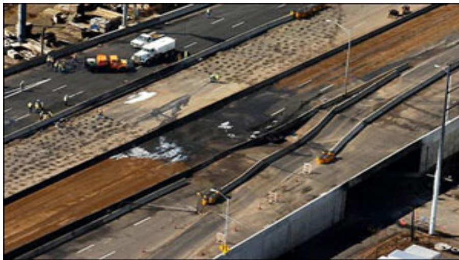
Figure 2.3b Buckling of I-95 Due to Tanker Fire.
