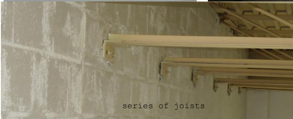
typical joist bearing with bottom chord extension
