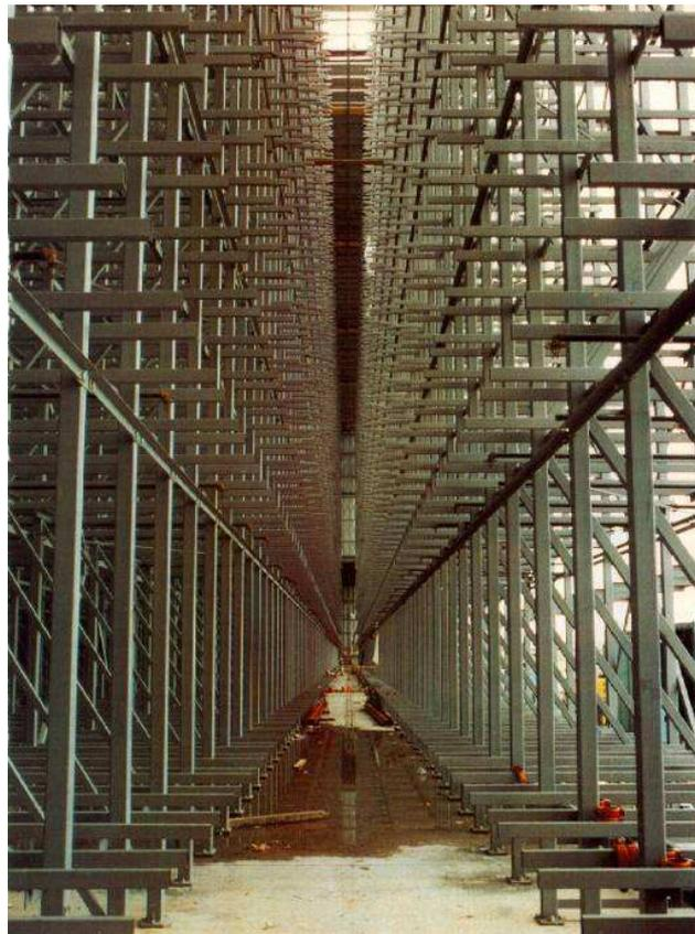
Rack structure, for automated retrieval of pallets
