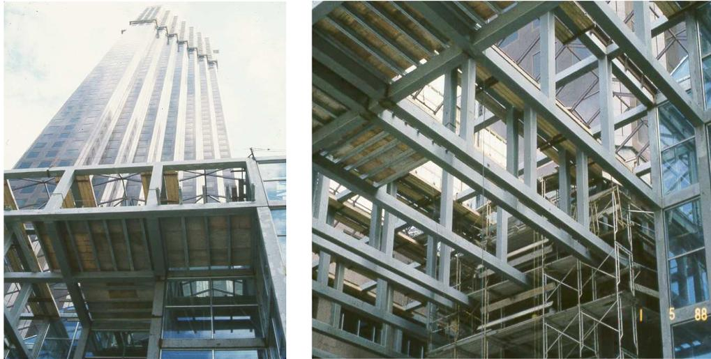
Figure 5.1 – Application of RHS Vierendeel trusses in the foyer of a building
