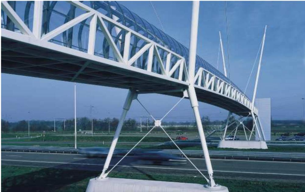
Figure 2.3 – Rectangular hollow sections used in a truss of a footbridge
