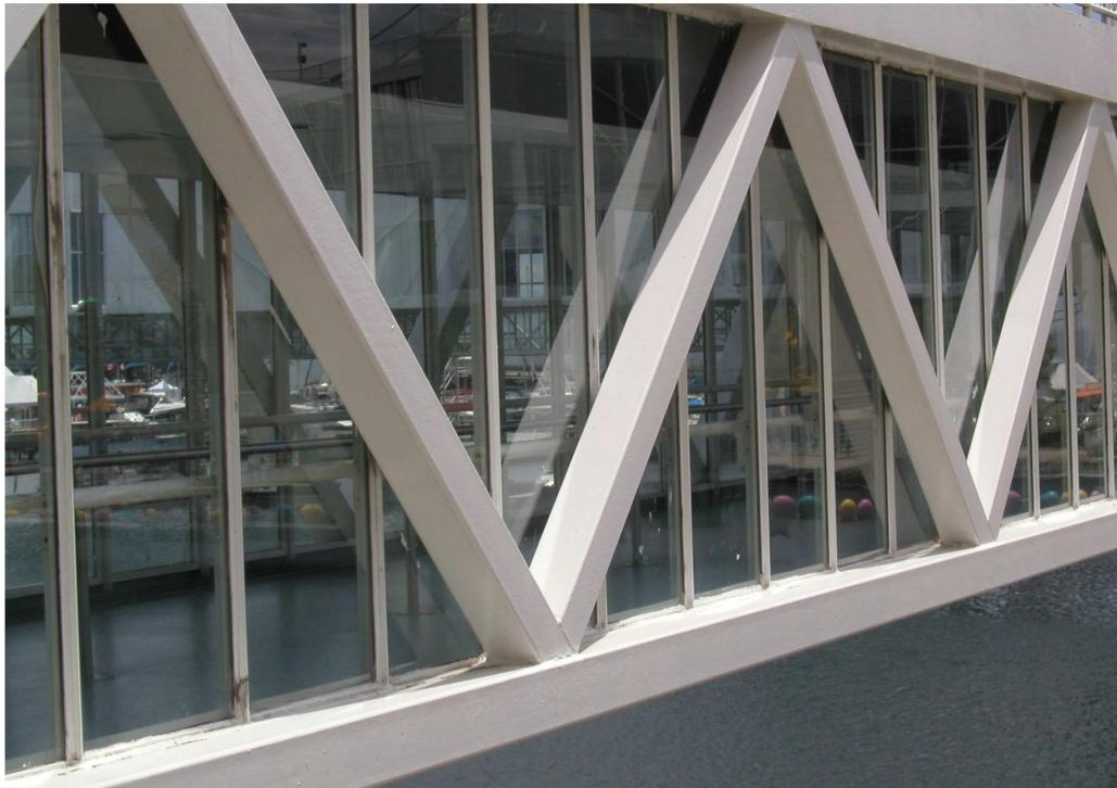
Truss with 100% overlapped joint
