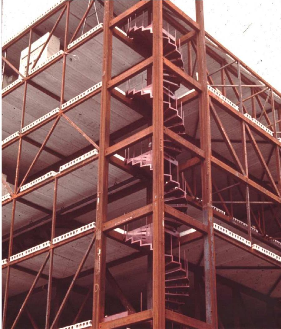
Figure 2.1 – Rectangular hollow sections used for the columns and trusses of a building
