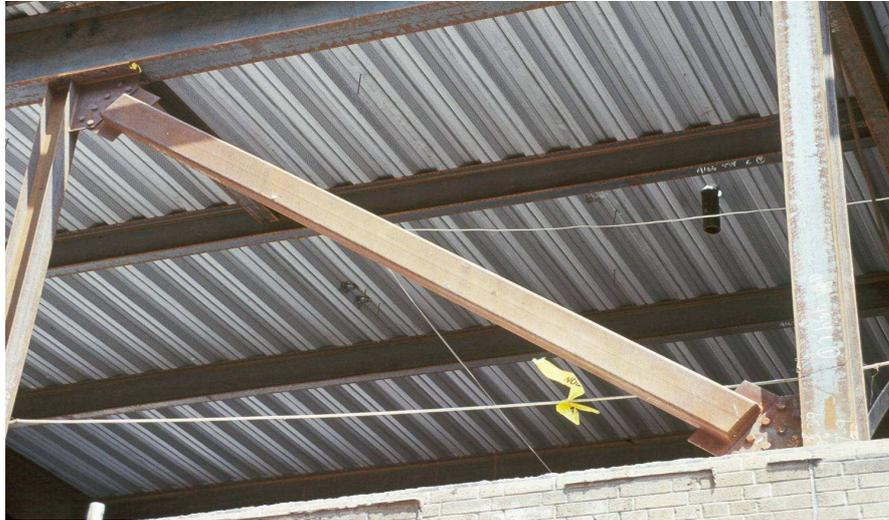
Figure 7.4 – Gusset plates slotted into a diagonal RHS bracing member, in a braced steel frame
