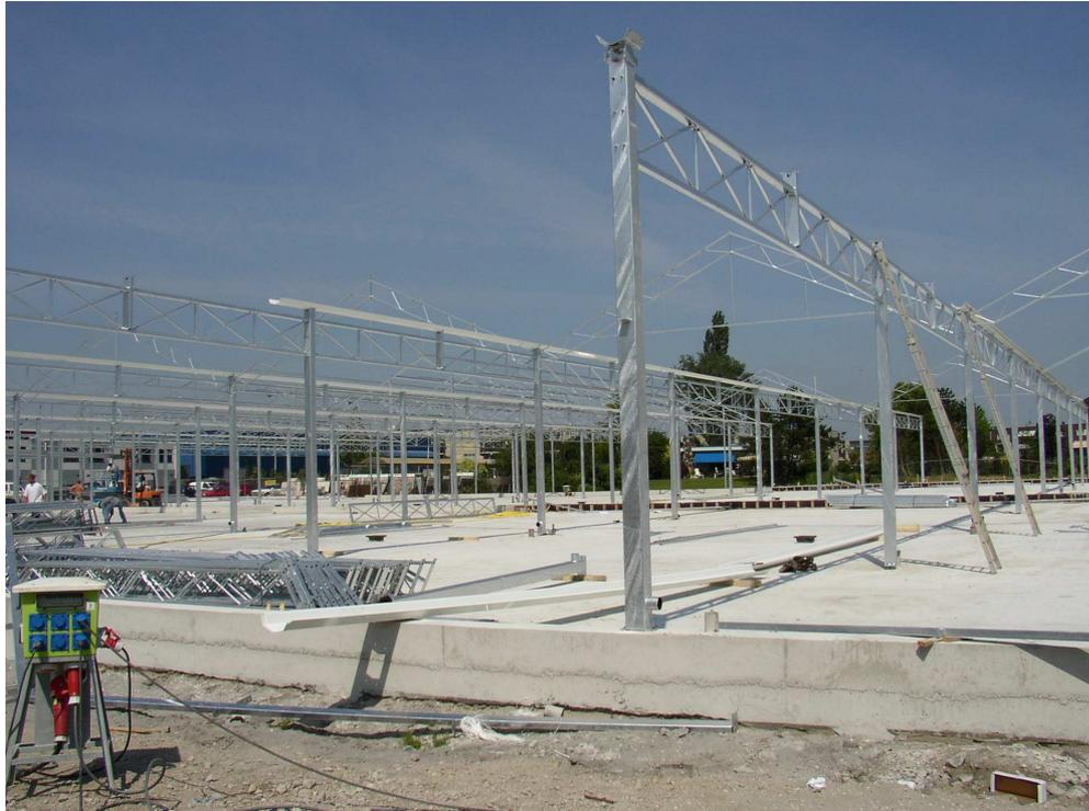
Figure 2.6 – Rectangular hollow section columns and trusses used in a glass house
