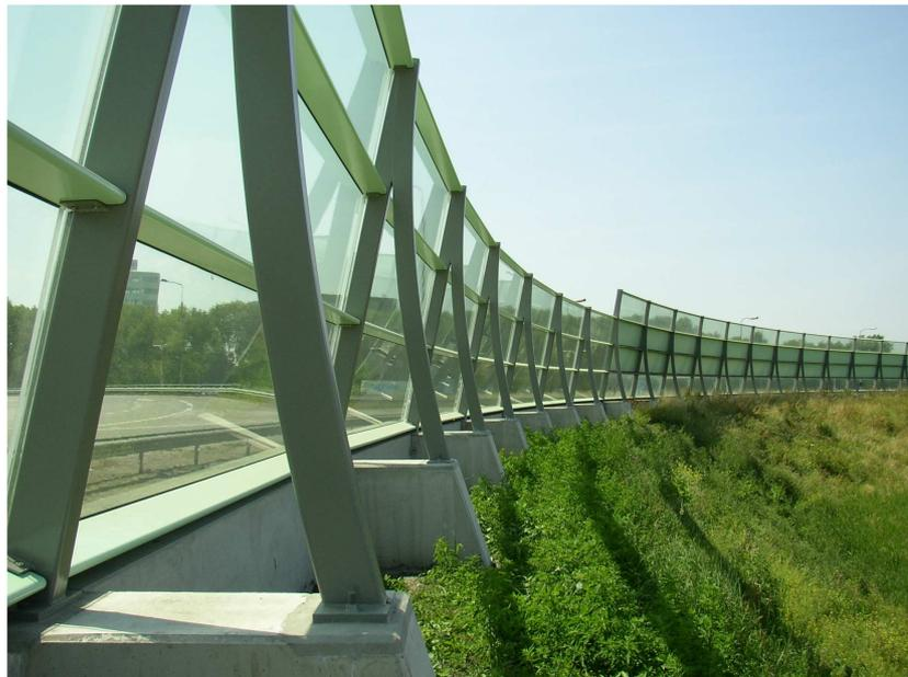
Figure 2.5 – Rectangular hollow sections used in sound barriers
