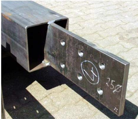
(a) Insertion of plate and welding to the RHS
