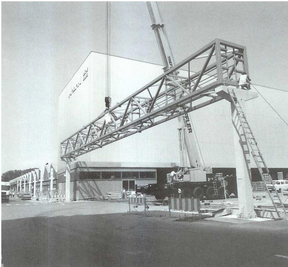
Erection of an RHS pipeline bridge
