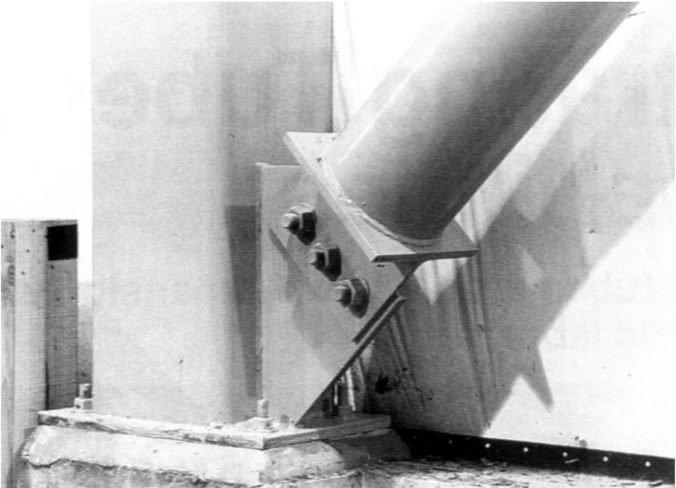
Figure 10.5 – Diagonal CHS bracing member connection to a RHS column via a longitudinal branch plate
