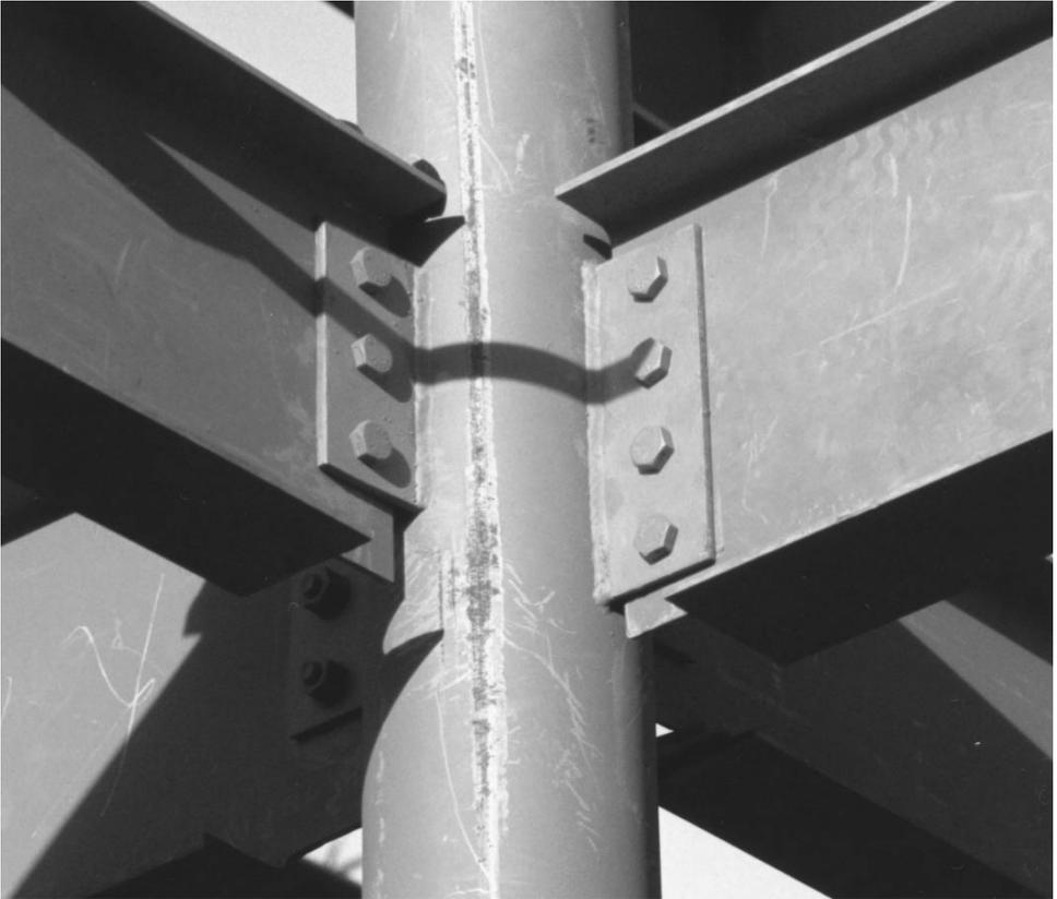
Figure 5.4 – Shear plate connection to CHS column
