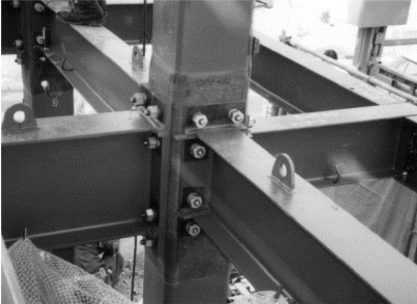
Figure 8.22 – End plate connection with blind bolts
