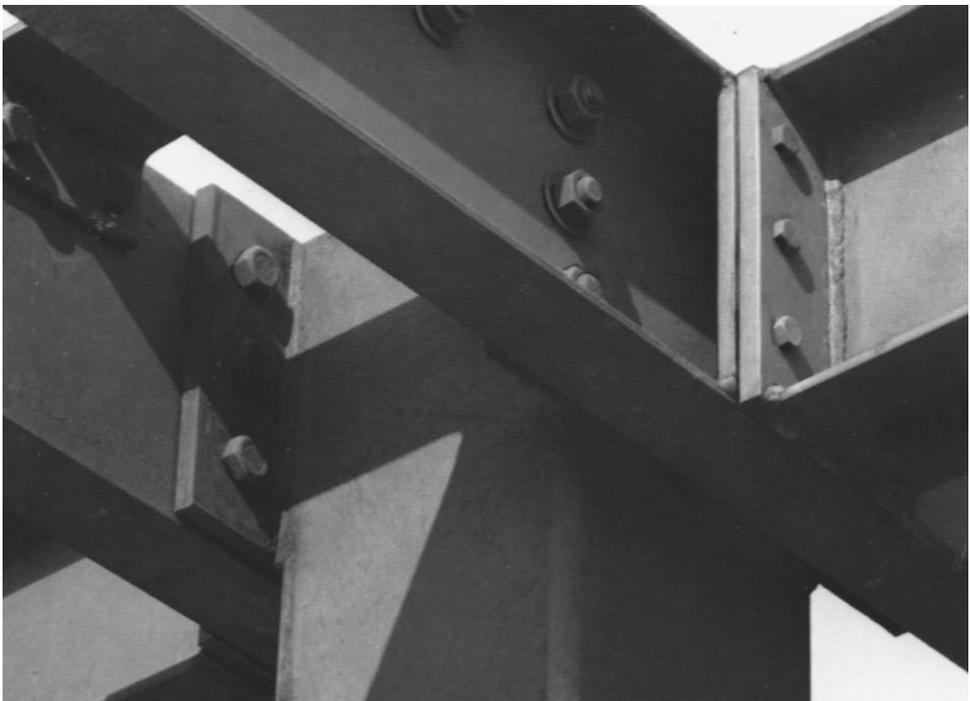
Figure 5.13 – Double channel beams bolted to plates on RHS column faces
