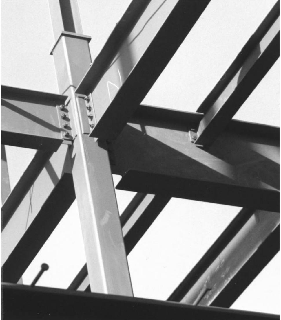
Figure 5.8 – Single angle connections to RHS column
