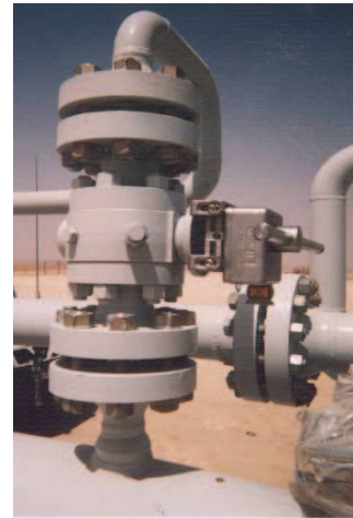
Ball valve with an Interlock installed
