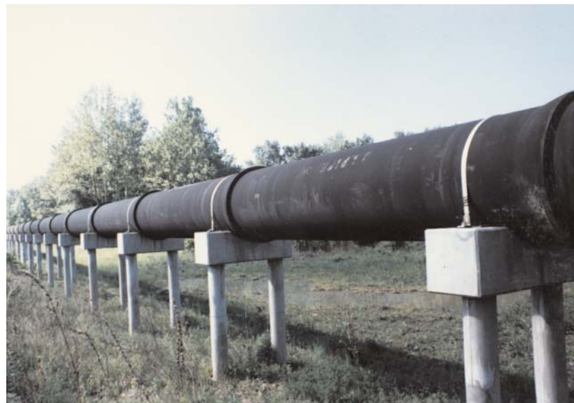
Ductile Iron is well-suited for use in pipe-on-supports applications due to its tremendous beam strength.
