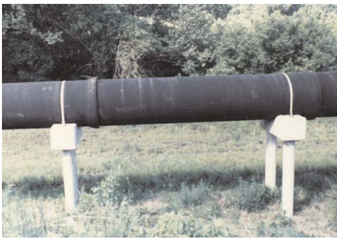
System security is maximized by positioning the supports immediately behind the pipe bells.
