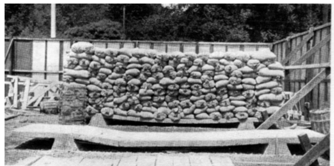
Test of Slab Reinforced with Clinton Electrically Welded Wire about 1915: In background, 4" slab, 1:2:4 concrete reinforced with Clinton Electrically Welded Wire, 3" x 12" mesh, No. 3 and No. 8 wires, giving area steel in longitudinal wires .187 sq. ins. per foot of width. Slab has center span of 12' with 3' cantilever at each end. In this view slab is loaded with 550 lbs. per square foot, but was subsequently loaded with 826 lbs. per square foot without failure. In foreground, slab of same dimensions, but reinforced with .18" sq. rods, 6'14" on centers, giving steel area .249 sq. ins. per foot of width. This slab failed with load of 486 lbs. per square foot.
