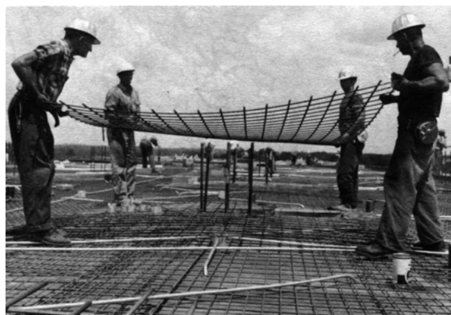
As industry grew, more and more flat sheets were used for structural fabric. These four men are positioning about 200 sq. ft. of reinforcement in one quick operation.
