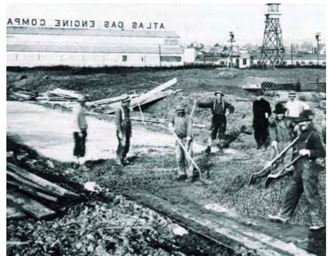
An early reinforced pavement built in 1913 at the Oakland, California waterfront. Compare the man hours here with today's high-production pavement.
