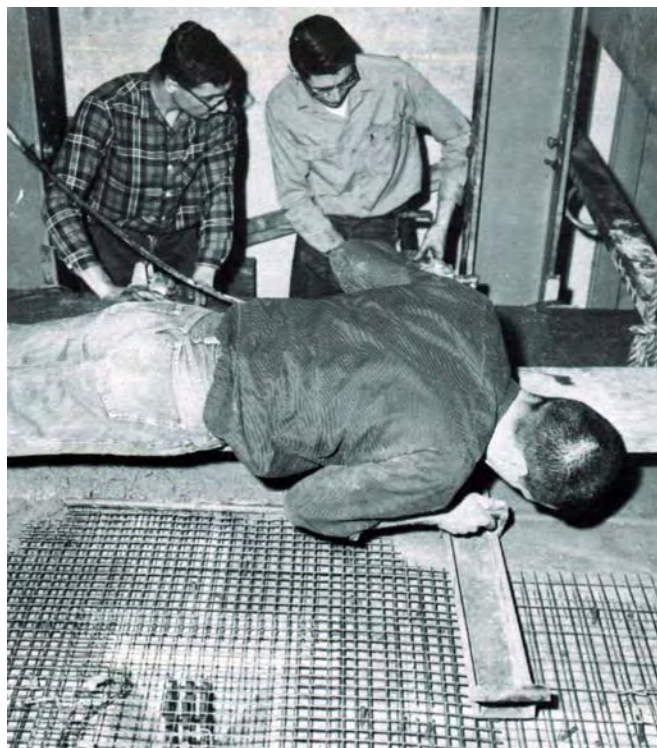
Graduate engineering students strike off and compact freshly placed concrete for 1314" thick flat slab test structure at the University of Illinois College of Civil Engineering Laboratory. Slab is reinforced by especially manufactured welded wire fabric reduced to quarter scale in size and spacing (see foreground). Test structure, 15 feet square, is a quarter scale representation of a 60-foot square slab supported by four interior columns.
