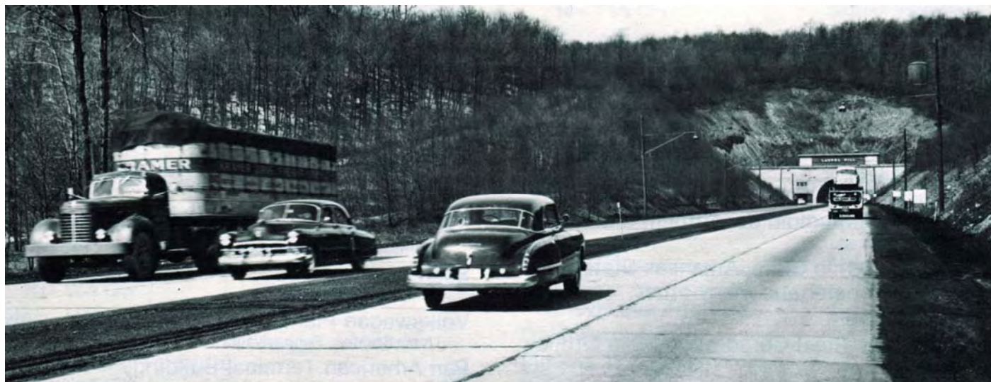
The Pennsylvania Turnpike is the granddaddy of the U.S. turnpikes and probably the Interstate System too. Its mesh-dowel pavement runs all the way from the Ohio line to Philadelphia and up to Scranton. We believe that this pavement was about 15 to 18 years old when this photo was taken.
