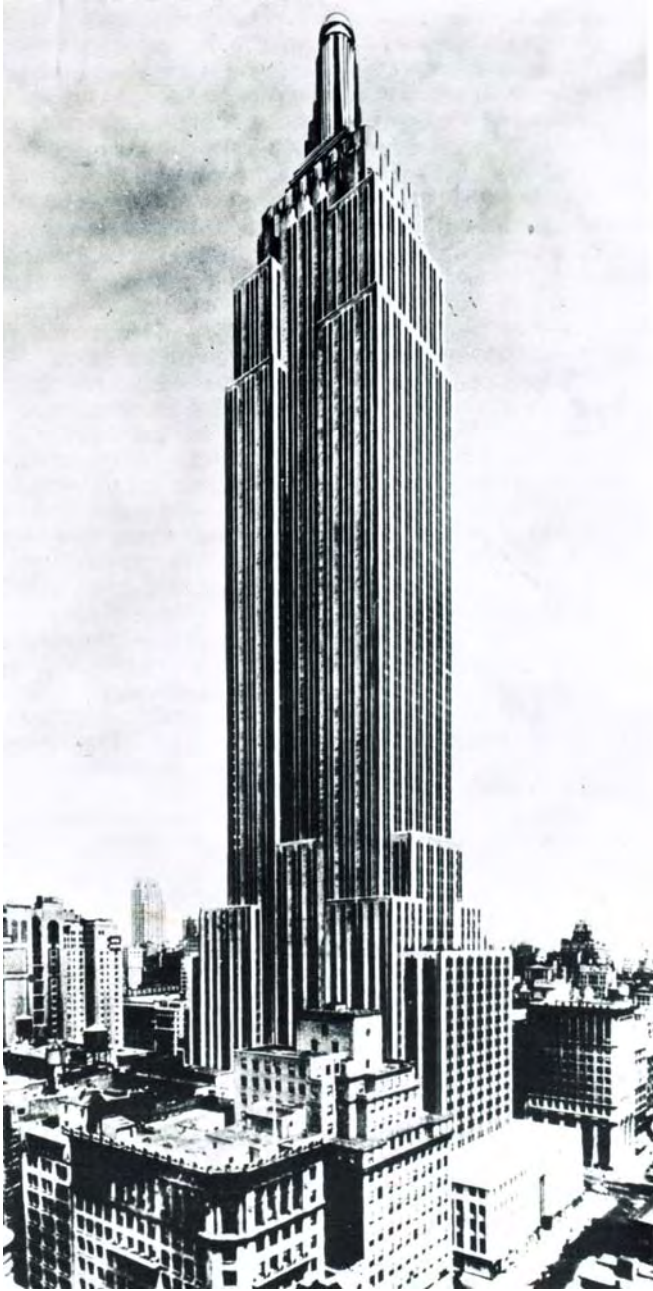
Fabric was widely used in Empire State Building-one of the world's most prestigious structures. All floor slabs used New York City's cinder arch construction method which required welded wire fabric.
