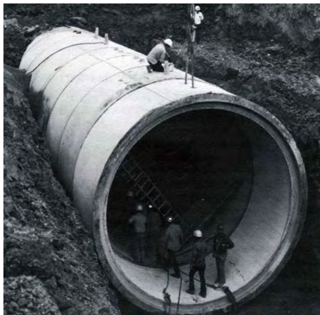
Concrete pipe in place. Inside diameter is 17 feet. Each section weighs 43 tons and required 4,000 lbs. of welded wire fabric.
