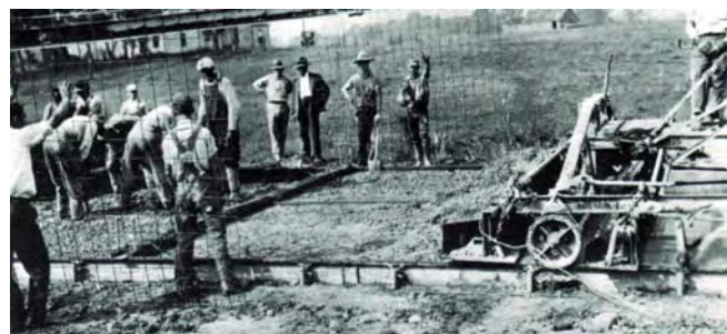
Midwest paving job. Placing WWF for Indiana highway, August, 1931.
