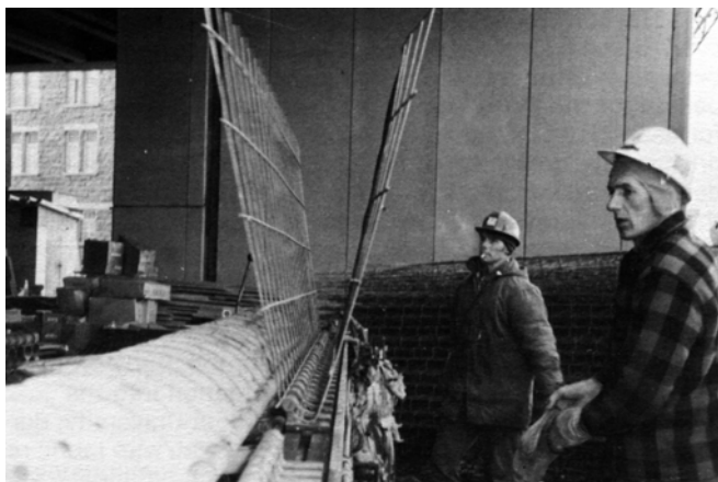
Bending equipment introduced by BSG became widely used in the 1970s and greatly expanded the use of fabric with the precast and prestressed industries and with contractors.
