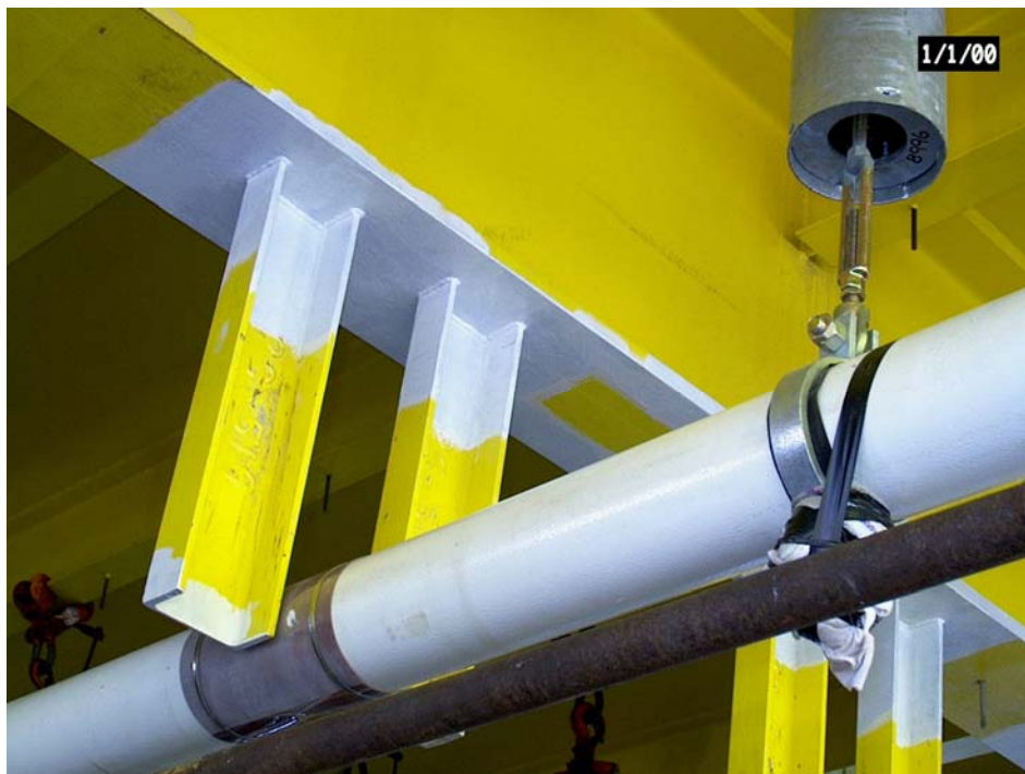
Figure 56 Type 7: Lateral support without vertical restraint
