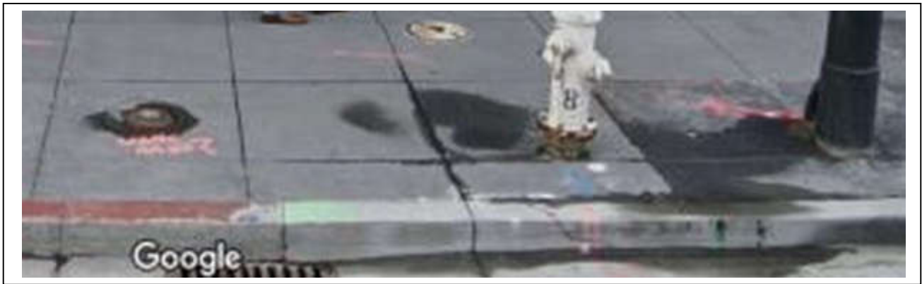
Figure 69: Close-up of the right side of Figure 67, showing the damaged concrete curb and groundwater seepage.
