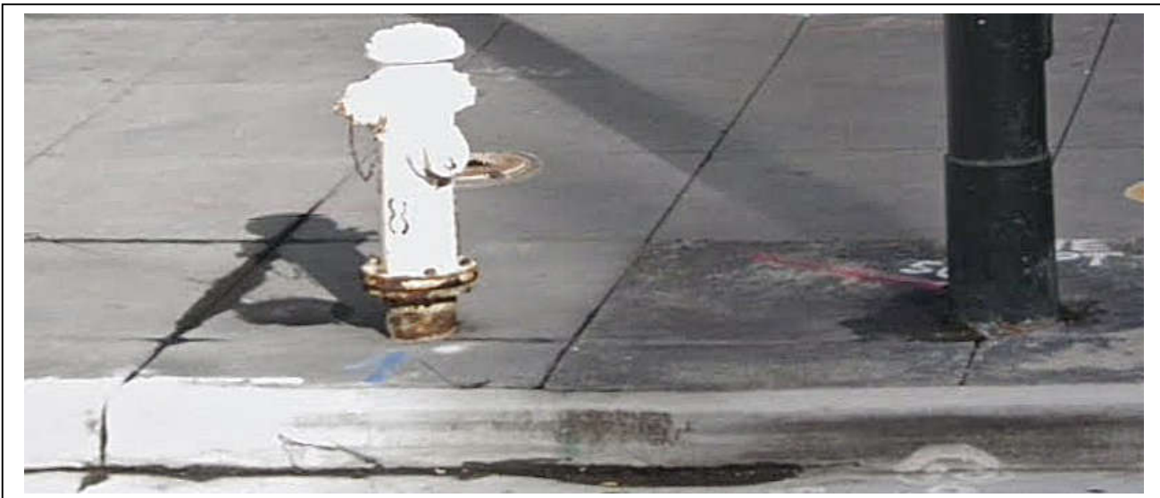
Figure 73: Close-up of the center of Figure 71, showing the damaged concrete curb and groundwater seepage.
