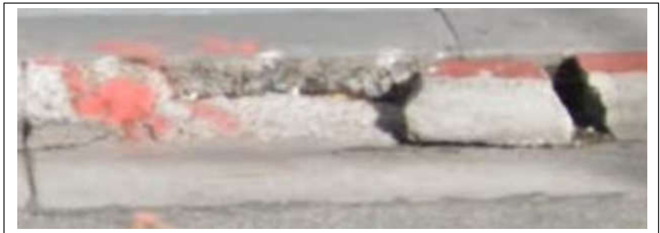
Figure 72: Close-up of the left side of Figure 71, showing the damaged concrete curb.
