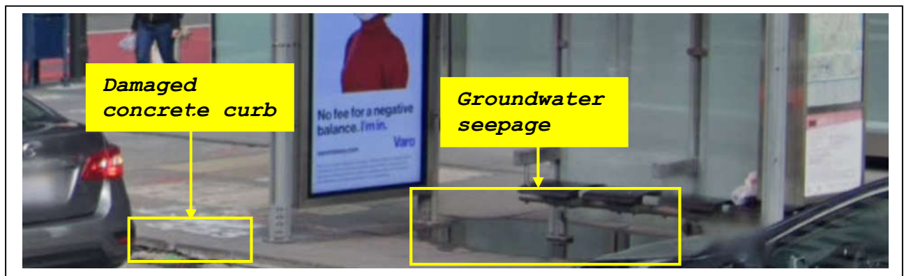
Figure 50: Close-up of groundwater seepage in Figure 49, viewed from a different angle.
