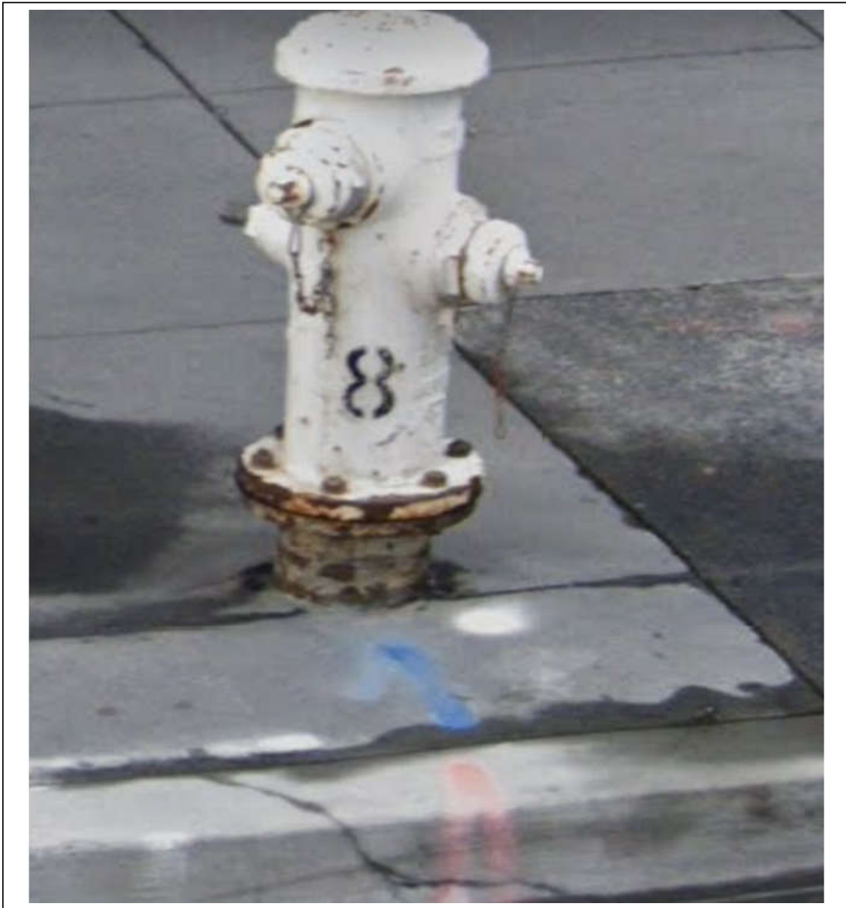
Figure 70: Close-up of Figure 69, showing the damaged concrete curb.
