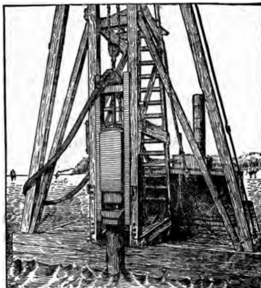
FIG. 33.—STEAM PILE-HAMMER IN OPERATION.
