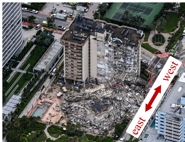
Fig. 1 Collapsed Champlain Towers South Condominium (photo via Agence France-Presse).
