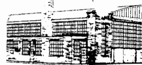
Fig. 3. Standard Form of Airplane Hangar—one story 'Leanto' along one side of building.
