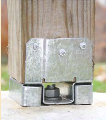
Figure 5. Frost footings do more than support the deck's downward load, they also anchor it against wind uplift. A positive hardware connection between the footing and the deck is needed.
