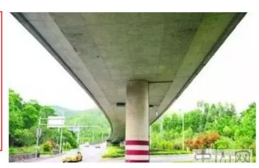
This bridge has enough curve for there to be a lateral load (as traffic drives in a curve, it pushes outward on the bridge deck).
