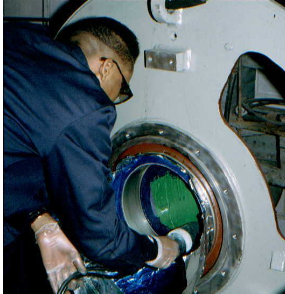
Figure 6.1: Example of using PVC sheet for masking.
