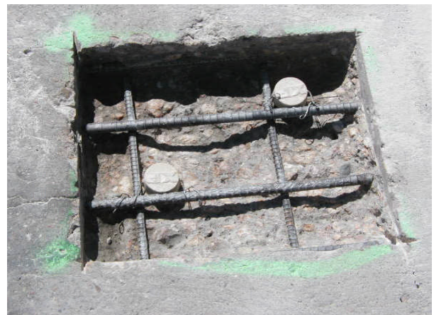
Galvashield® XP+ anode (above) Euclid Sentinel-GL (below)
