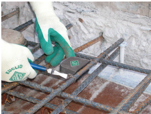
Galvashield® XP+ anode (above) Euclid Sentinel-GL (below)
