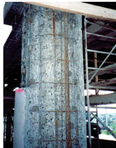
Galvashield® XP+ anode (above) Euclid Sentinel-GL (below)
