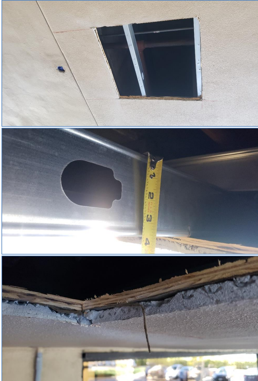
Figure 6: Hung soffit exploratory work and MC documentation of conditions.
