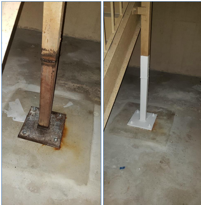
Figure 3: Column base repair.
