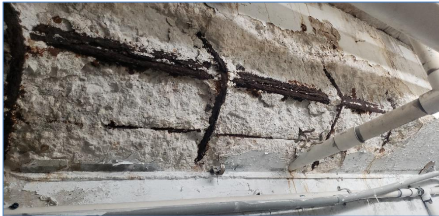
Figure 1: Loose, cracked, spalled deteriorated concrete removed at pool corbel, Pool Pump Room.
