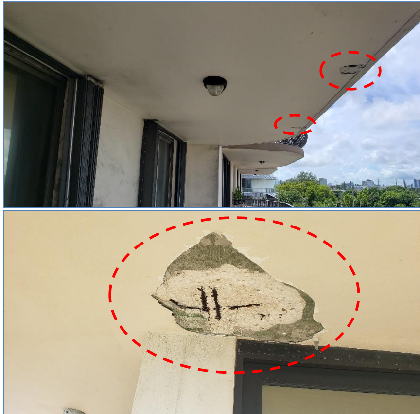
Figure 8: Balcony soffit concrete and stucco removal by CPR.
