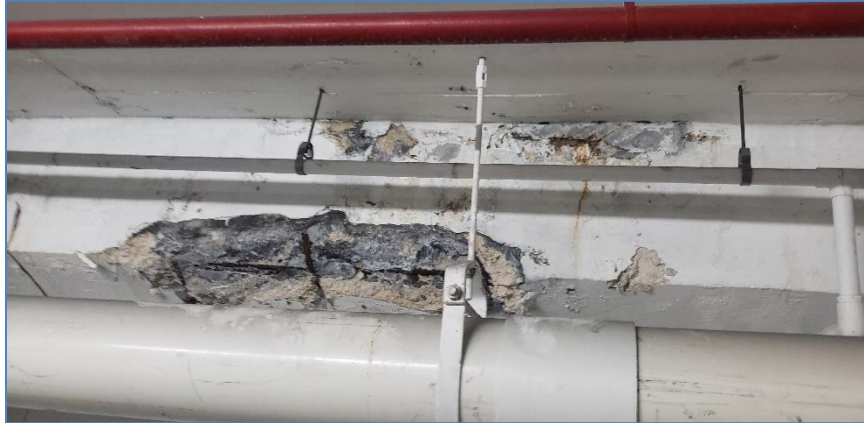
Figure 2: Loose, cracked, spalled deteriorated concrete removed at pool corbel, pool perimeter.
