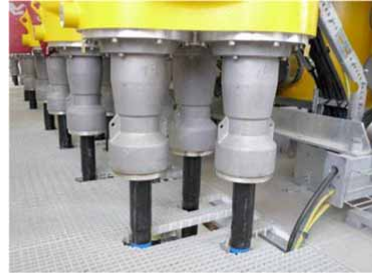
72 kV plug-in cable terminations
