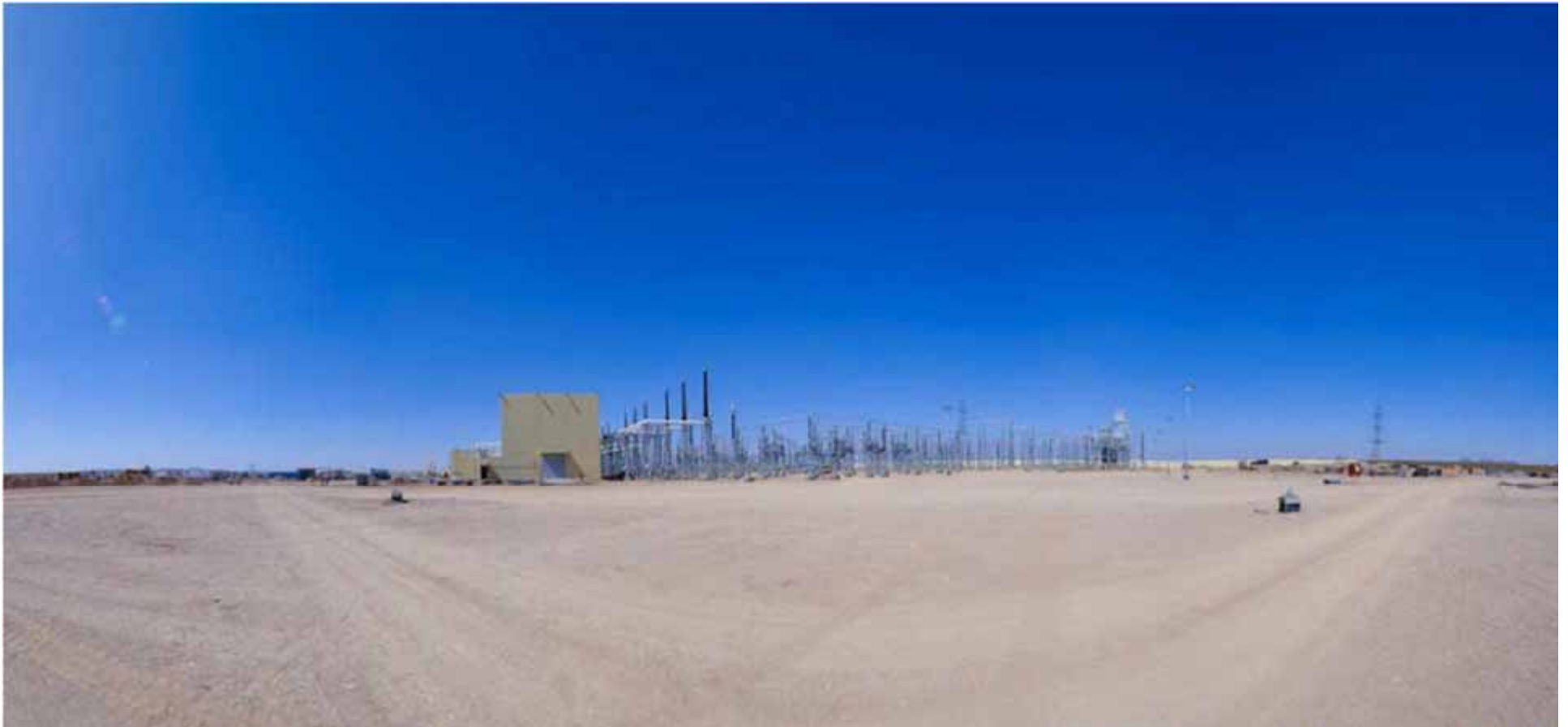
Saudi Arabia - Qassim - 420kV Outdoor temperature up to +55°C
