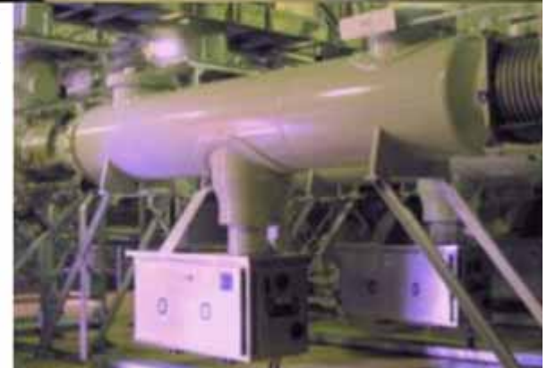
Canada - Mica - 550 kV - old 6-breaks CB replaced by 2-breaks modern CB
