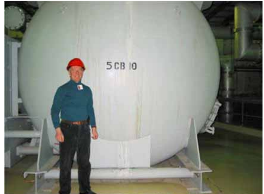
Canada - Mica - 550 kV - old 6-breaks CB replaced by 2-breaks modern CB
