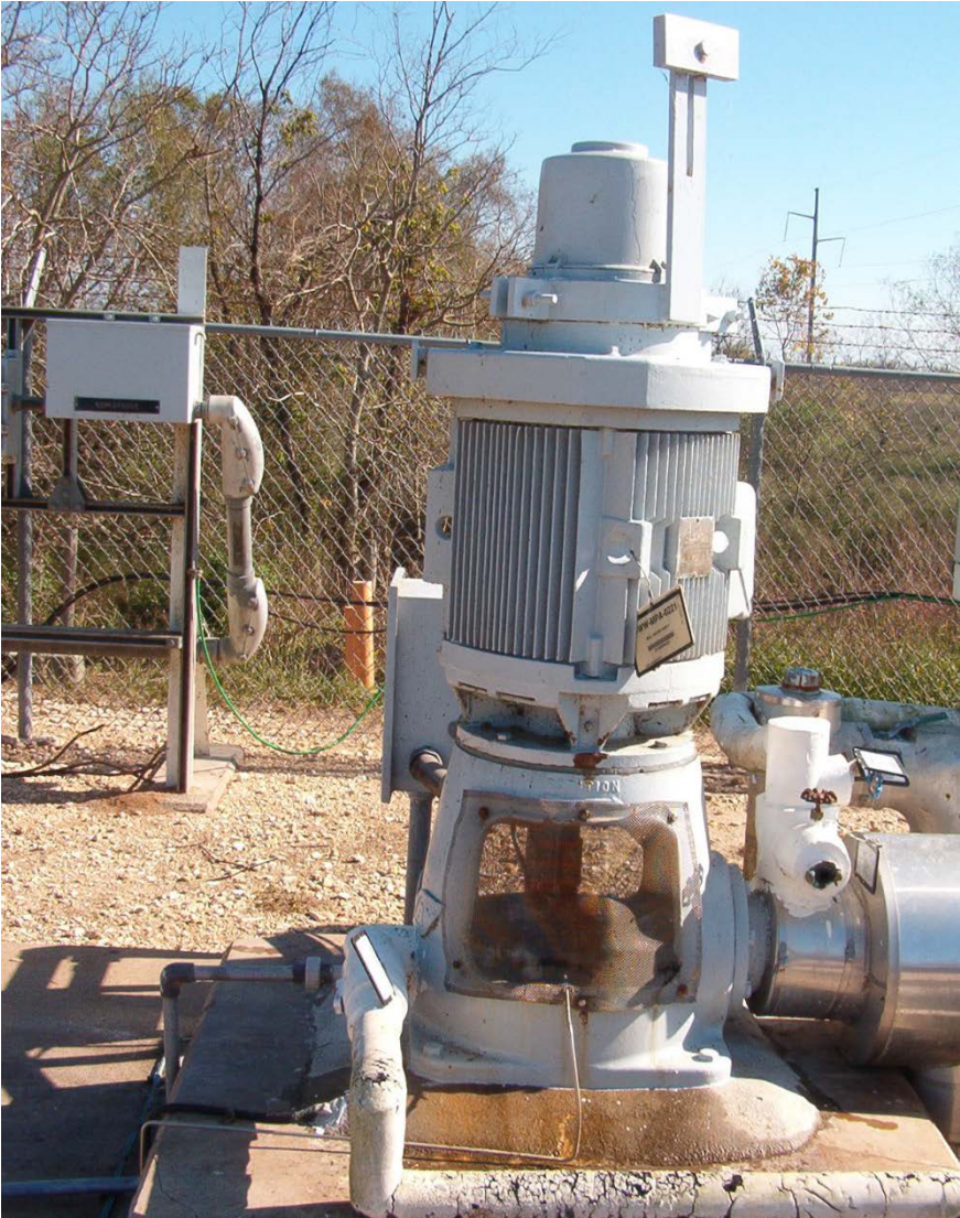
Clamp – eliminated the need to Drill/weld on the machine itself
