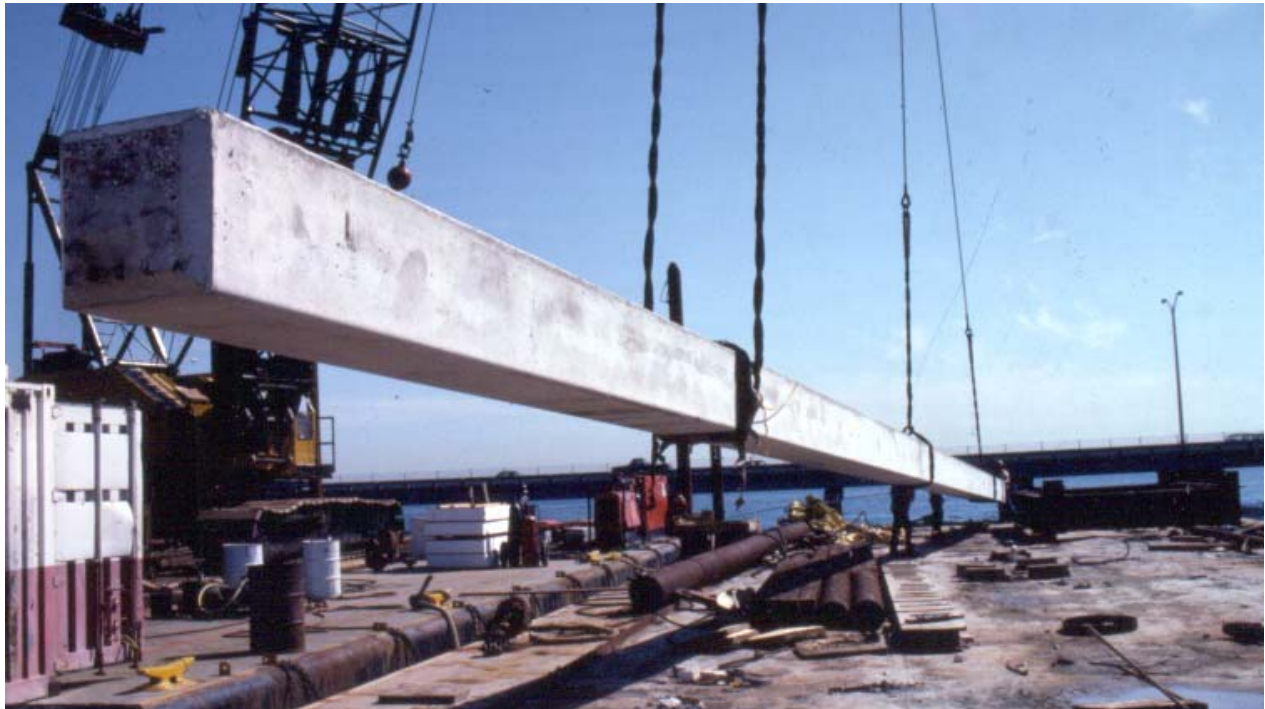
Figure 8.8 Square Prestressed Concrete Pile
