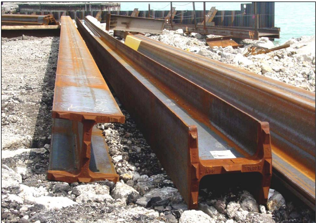
Figure 8.3 H-piles with Driving Shoes
