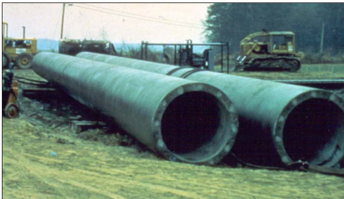
Figure 8.11 Concrete Cylinder Pile
