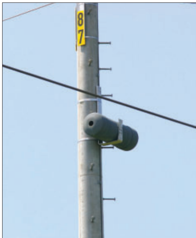
FIGURE 6.19: Kestrel nesting tube (91-cm [36-in] length) installed on transmission tower in Georgia.
