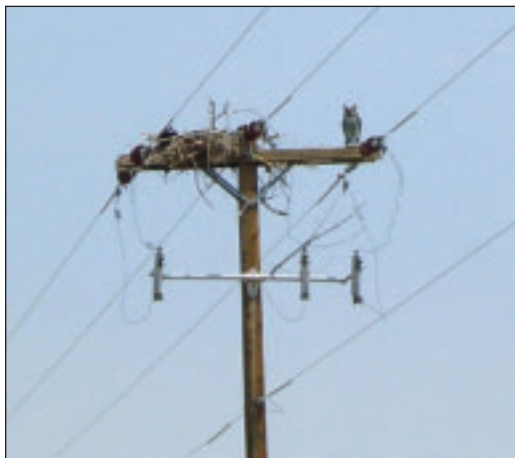
FIGURE 6.26: Osprey nest constructed on pole with plastic owl intended to haze birds.
