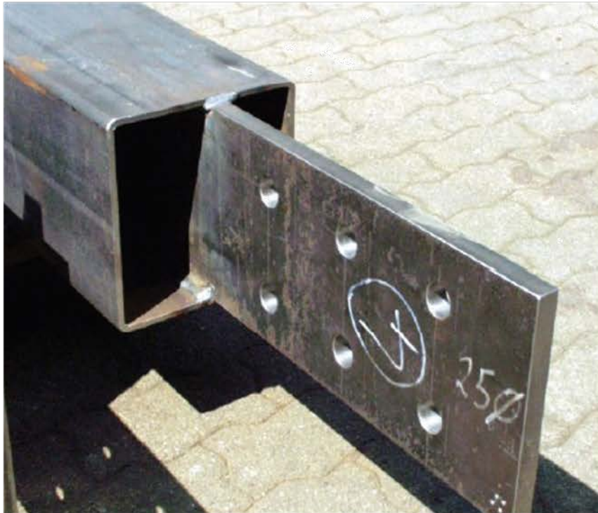
FIG. 4-1.19 HIDDEN BOLTED CONNECTIONS – PACKER (2016)
