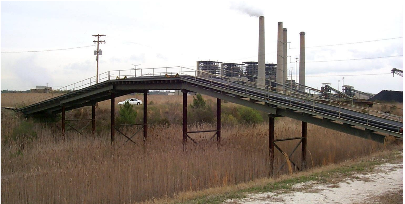
Pipe Bridge for Polyethylene Lines Over Active Railroad Spur
