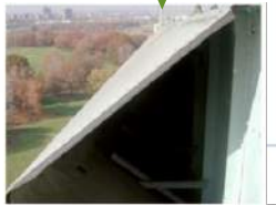
The wedge shaped wind fairing used on the Bronx-Whitestone Bridge
