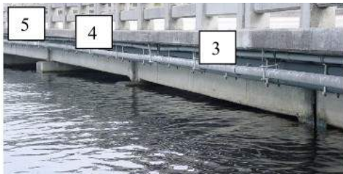
Report: BDV31 977-01 (University Blvd Bridge, 2011)
