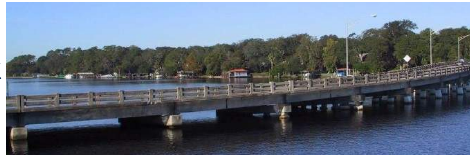
Figure 131—University Boulevard Bridge
