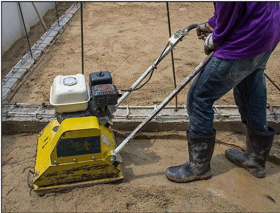
Figure 1 - Plate compactor in use on residential site
