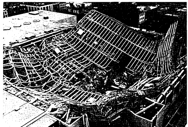
FIG. 1. Hartford Civic Center Coliseum Roof Collapse, 1978 (Construction Failure, Feld and Carper, © 1997. Reprinted by Permission of John Wiley & Sons, Inc.)
