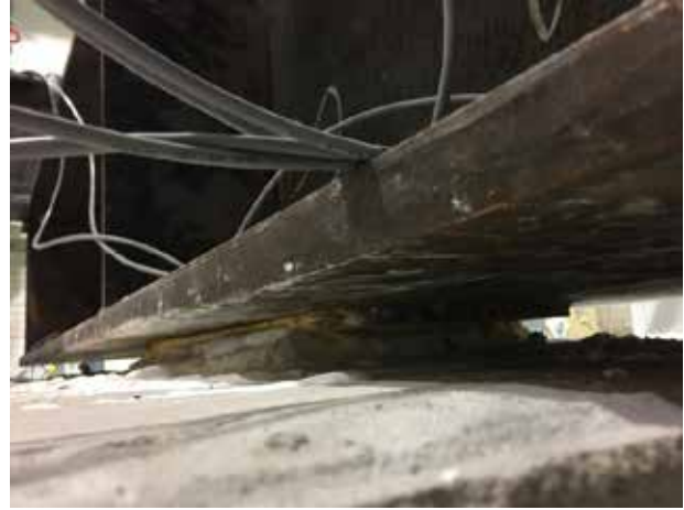
(b) Steel Plate and Gypsum Cement between Loading Frame and Specimen
