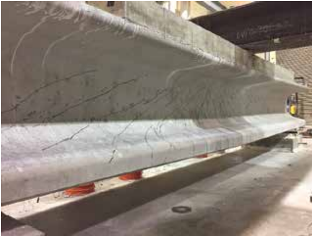
(a) Cracking at 400 kips
