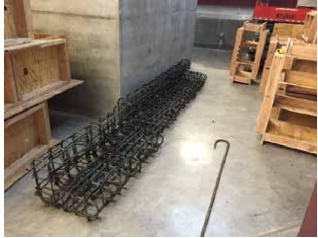
(b) Reinforcement Cages
