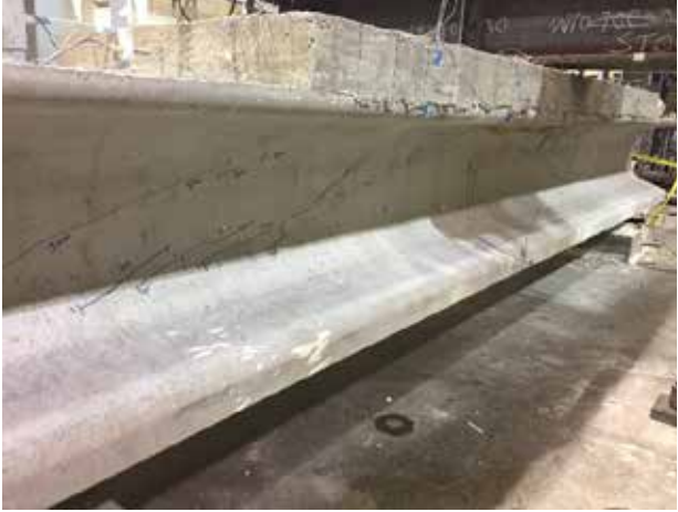
(a) Web Shear Cracks at 205 kip
