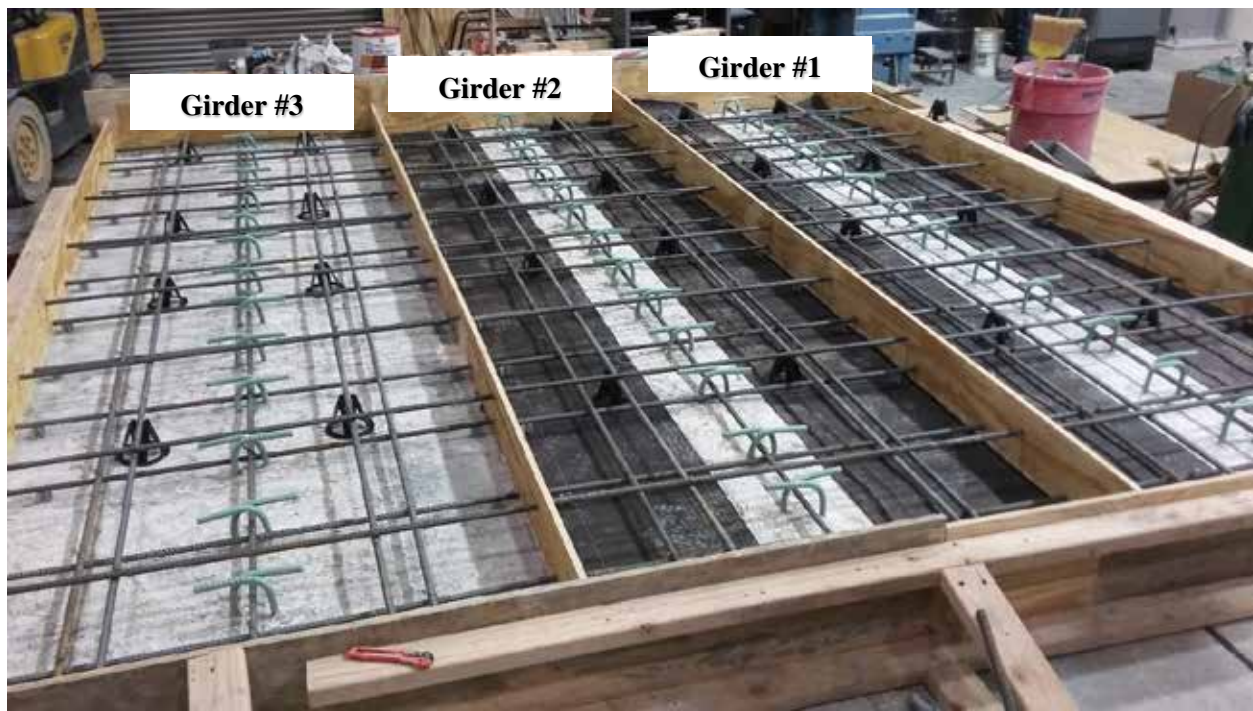
Figure 4.15: Surface Preparation and Deck Reinforcement before Casting
