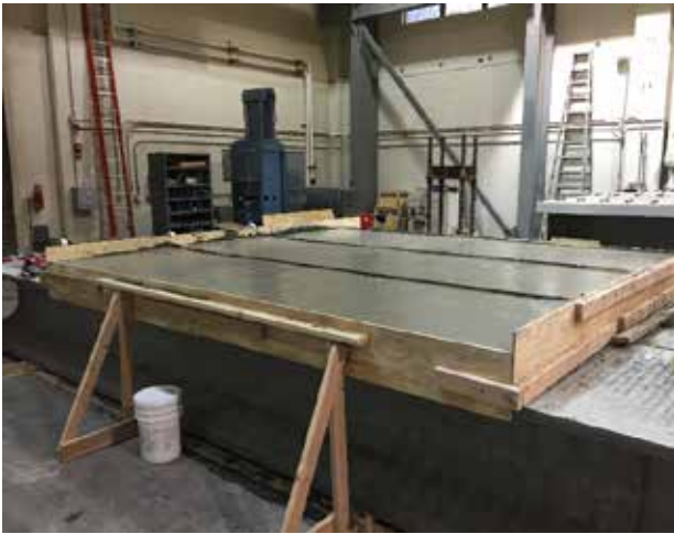
(b) Concrete Deck after Finishing
