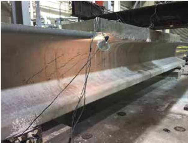
(a) Cracking at 300 kips
