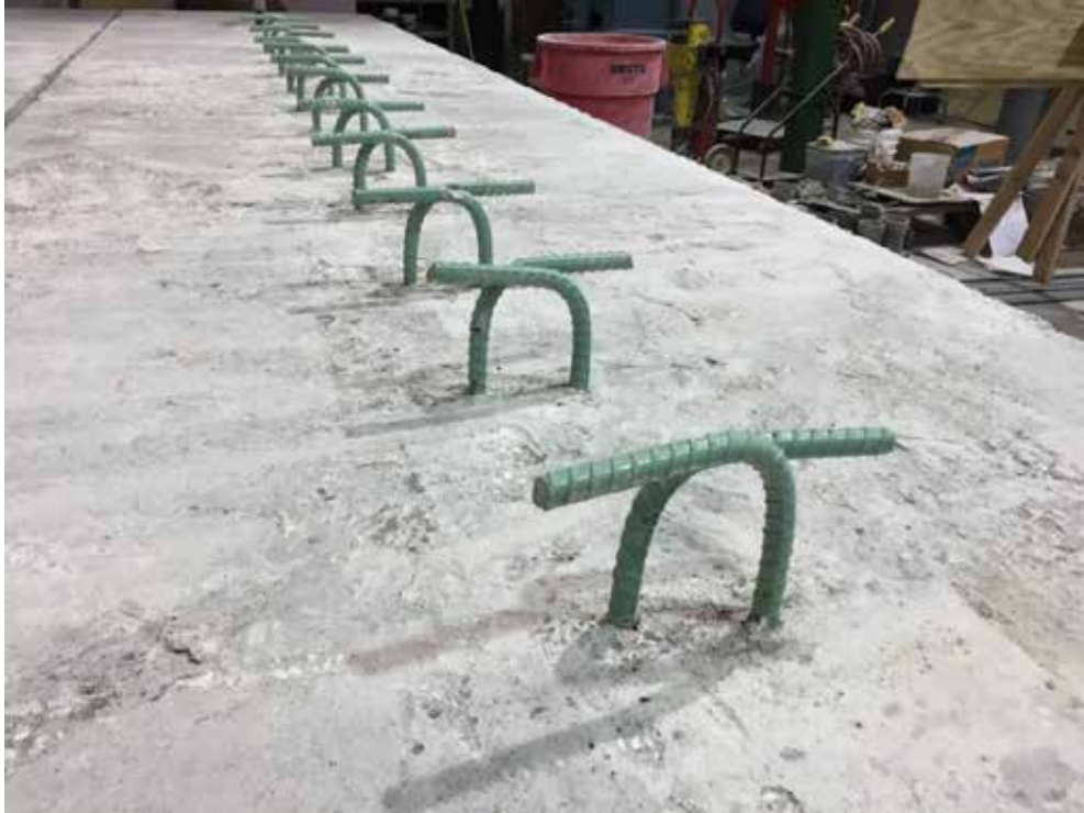
Figure 4.14: Girder #1 Surface after Deck Removal (Originally Fully Troweled)
