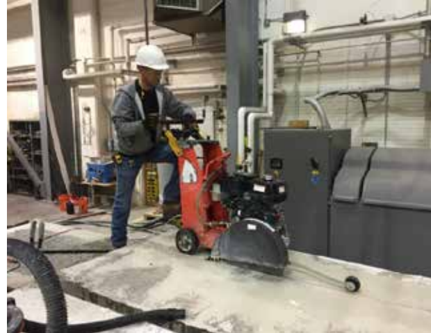
(b) Longitudinal Saw-Cuts
