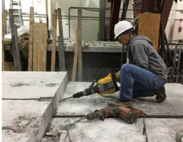
(b) Use of Demolition Hammer at a Low Angle to Break Deck Sections Free
