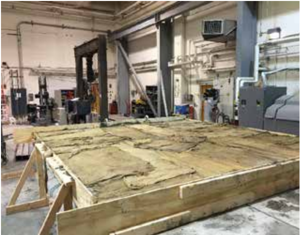
(c) Concrete Deck Curing
