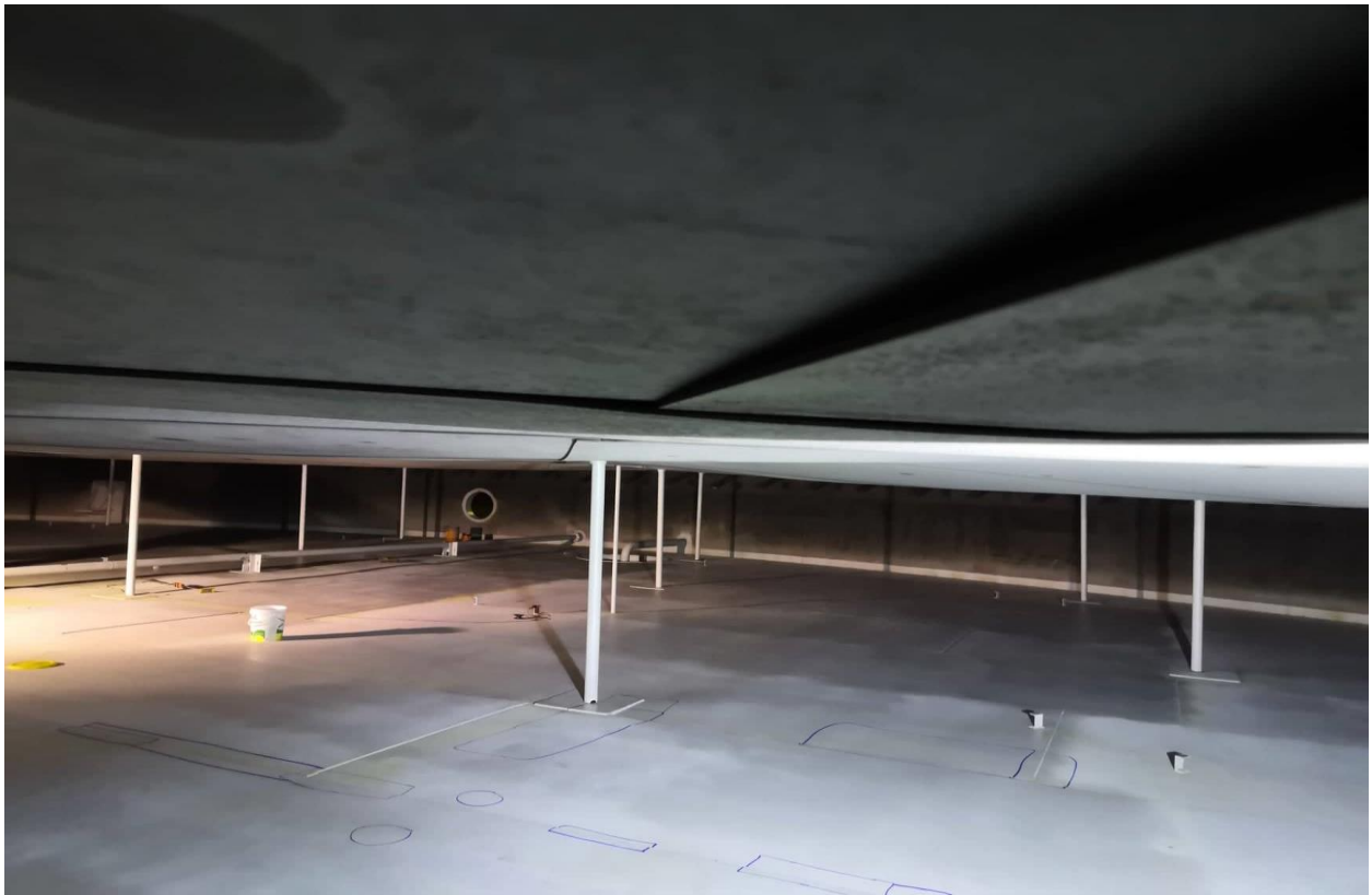
Roof Deformation and an inclined leg support
