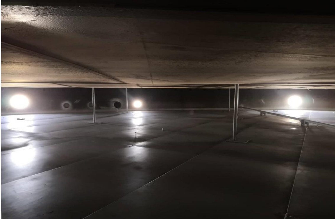
Roof Deformation and an inclined leg support
