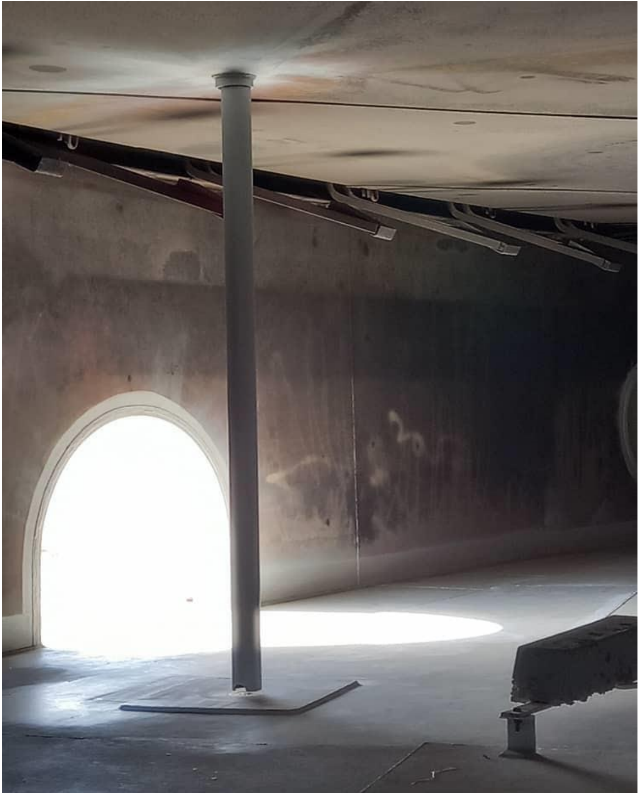
Clearance between the leg support and its bottom pad
