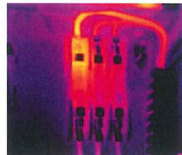
*An overheating terminal in an industrial fuse block. By Hotflashhome (Own work) [CC BY-SA 3.0 (<http://creativecommons.org/licenses/by-sa/3.0>) or GFDL (<http://www.gnu.org/copyleft/fdl.html>)], via Wikimedia Commons*
