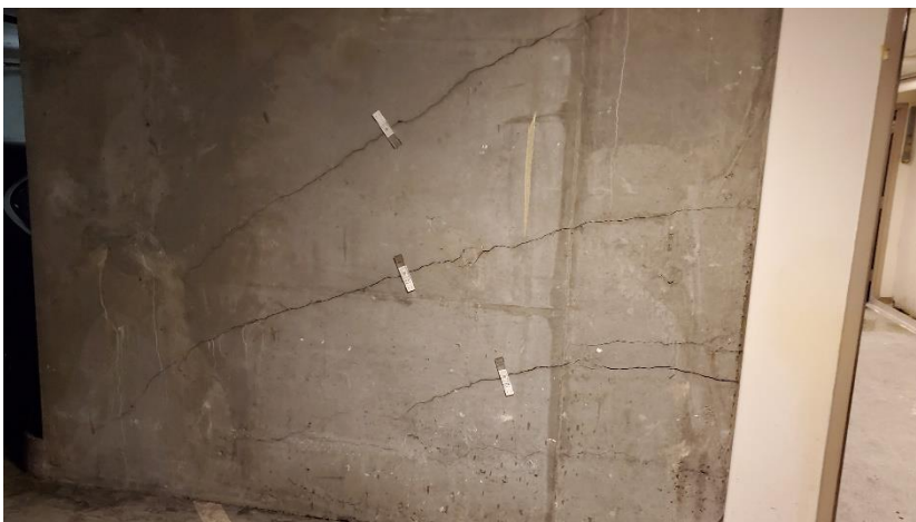
Photo 11 Podium shear wall at level B1
