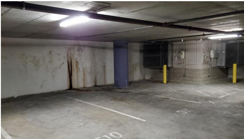
Photo 13 Podium north basement wall at level B1
