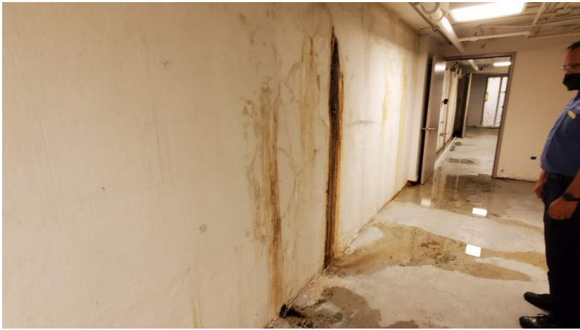
Photo 6 Podium west basement wall at level B1
