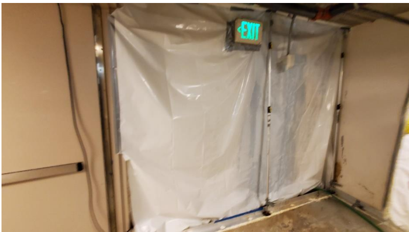
Photo 8 Podium west basement wall at level B1
