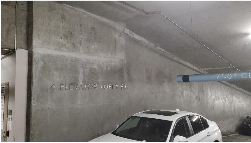
Photo 18 Interior podium ramp shear wall at B1
