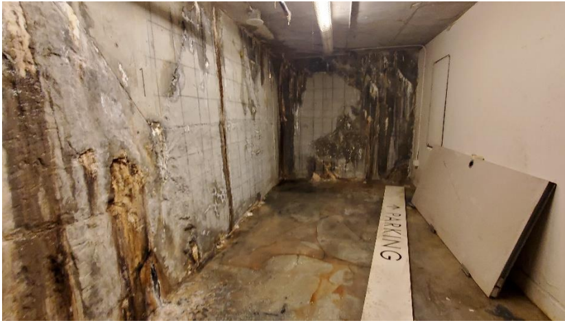
Photo 9 Podium west basement wall at level B1
