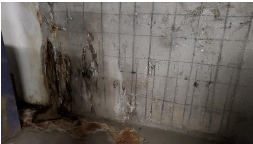
Photo 14 Podium east basement wall at level B1
