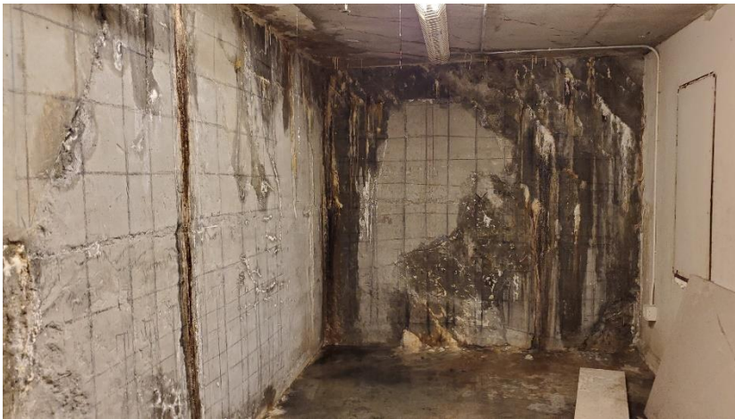
Photo 10 Podium west basement wall at level B1
