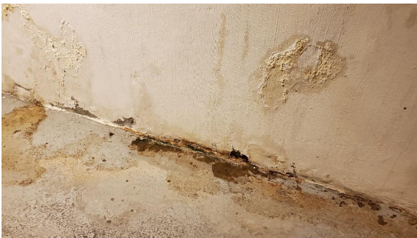
Photo 2 Podium west basement wall at level B5
