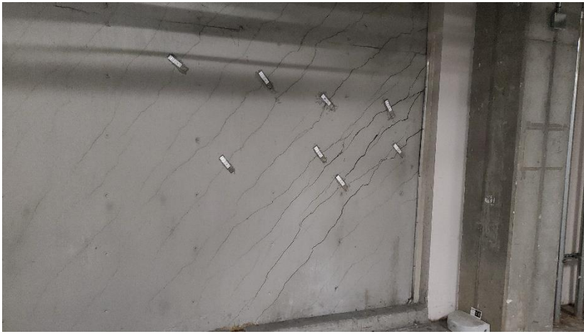
Photo 15 Podium east basement wall at level B1
