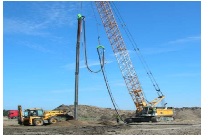
Figure 1. Vibro Concrete Column
