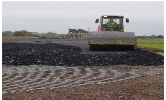
Figure 2. Steel Reinforcement Cage under Embankment – LGV Project Paris - Bordeaux
