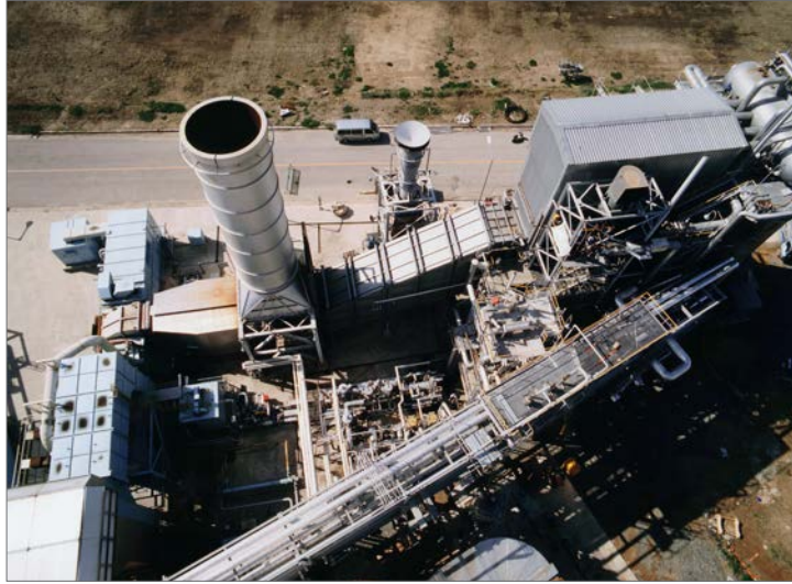
Figure 13: High hydrogen fueled 6B.03 gas turbine.
