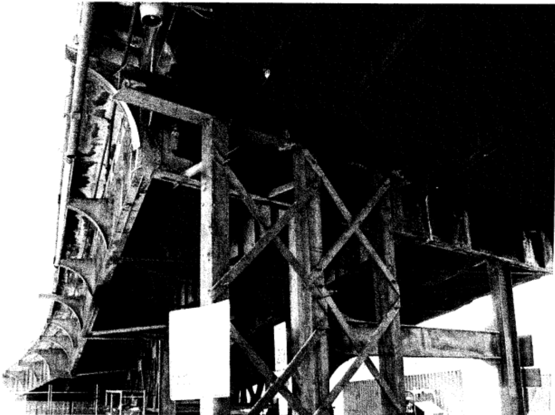
Typical View of Steel Bent Cap
