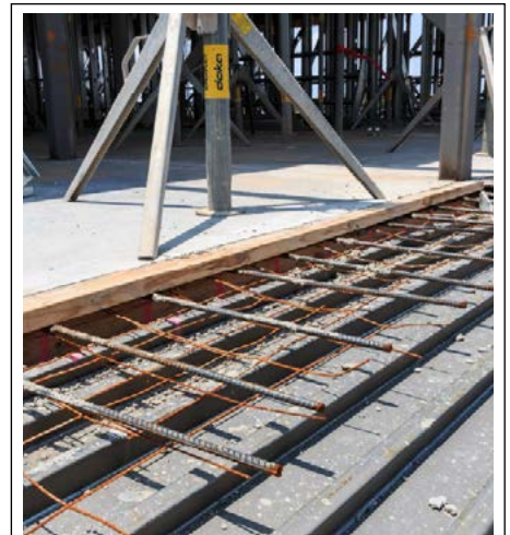
CONCRETE CONSTRUCTION JOINT
