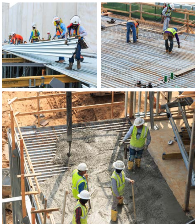
Deck installation, slab reinforcement placement and concrete casting incorporate traditional equipment and methods.
