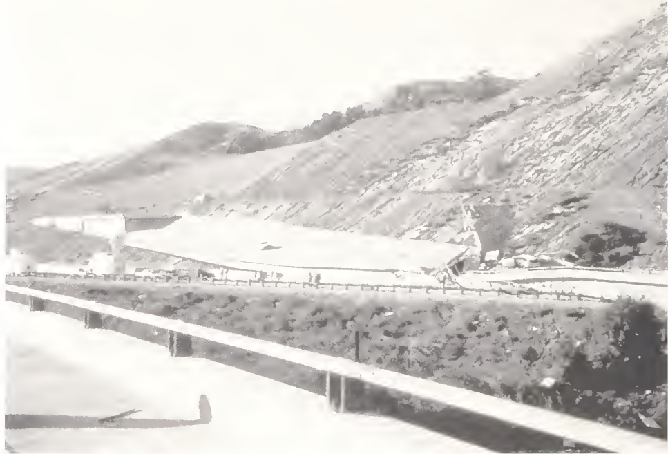
Figure 4.11. Overview of the collapse of the SR14/I5 Separation and Overhead, Ramp C, looking to the south at Abutment 1. Pier 3 can be seen at the right of the photograph (Photo courtesy of EERC).
