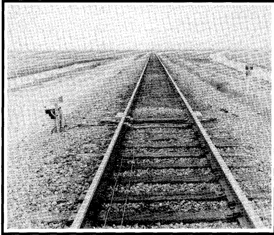
Figure 8. Acoustic Receivers of a Wayside ABD Installation
