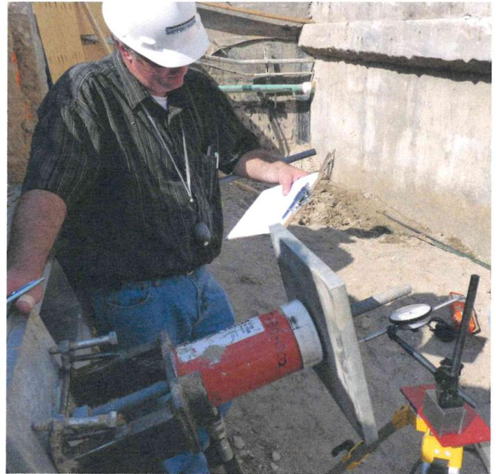
*Pretensioning a Helical Tieback*
