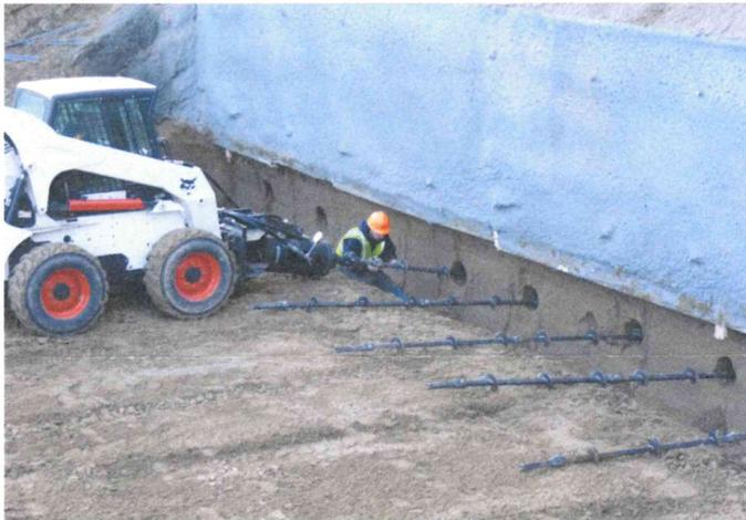
Installation of helical soil nails
