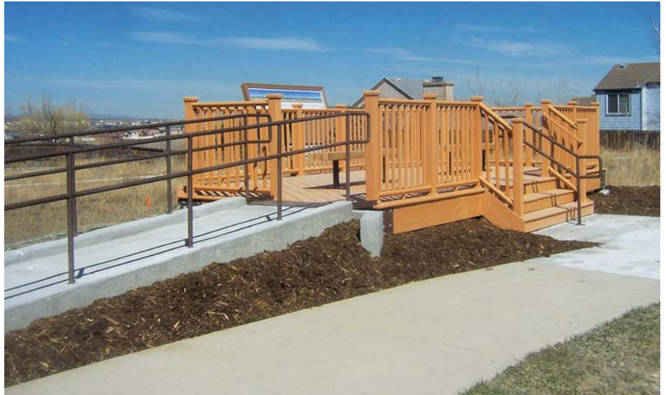
Figure 1. Even small public decks such as this view platform must have at least one accessible egress path.
