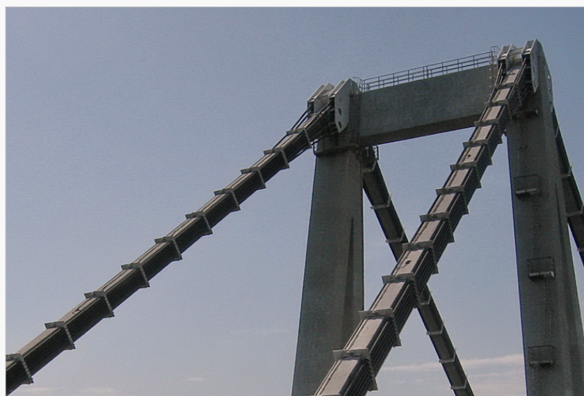
Pylon 11: External reinforcement cables installed 1992-1994. (Hasen 2007)
